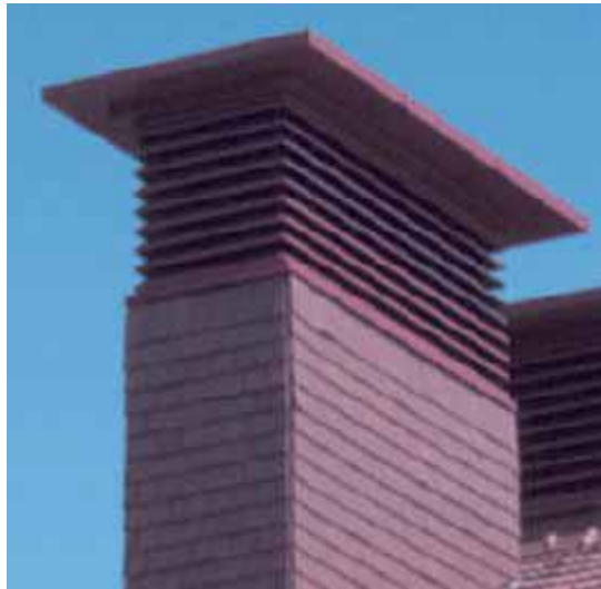
Fig 2.18 Louvered Penthouse [20]
