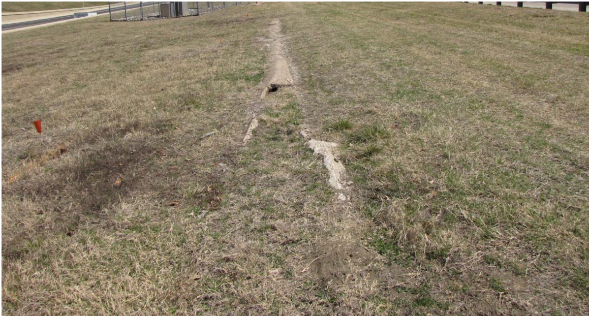
Figure 3-15: Abandoned Utility in the Retained Zone
