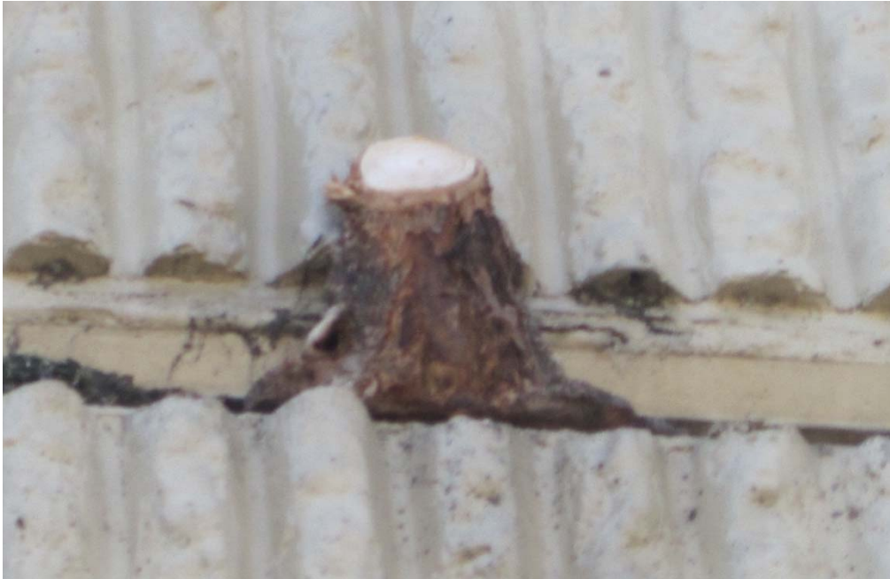
Figure 3-8: Tree Growth Through Panel Joint
