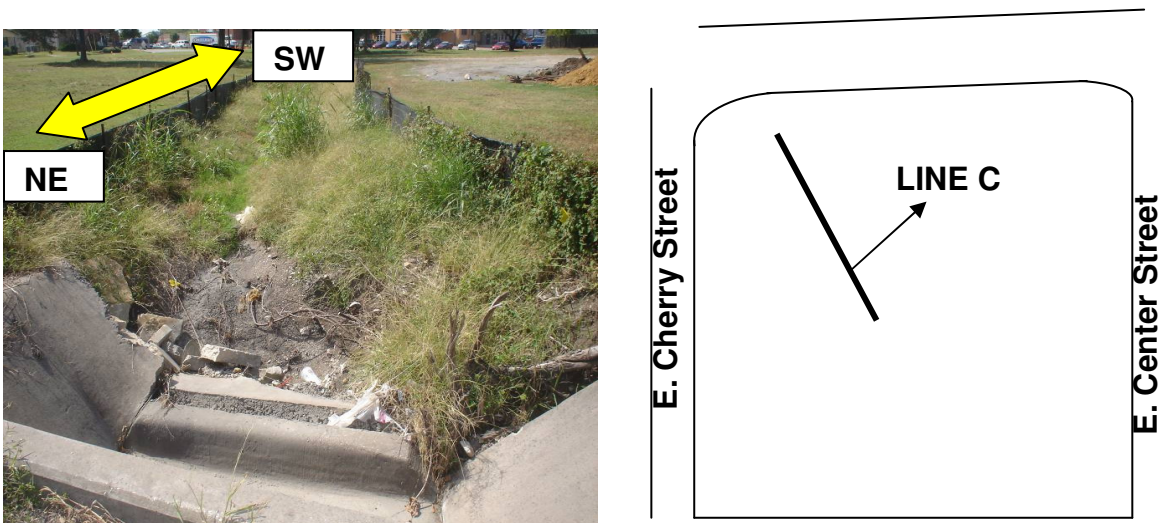
Figure 3.15: Line C survey along the channel
