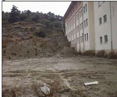
Figure 2.18: Study area after the landslide (Drahor, 2006)
