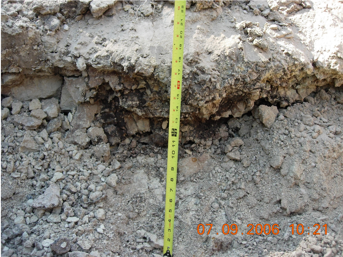
Figure 3.9 Organic rich zone in subgrade soil.
