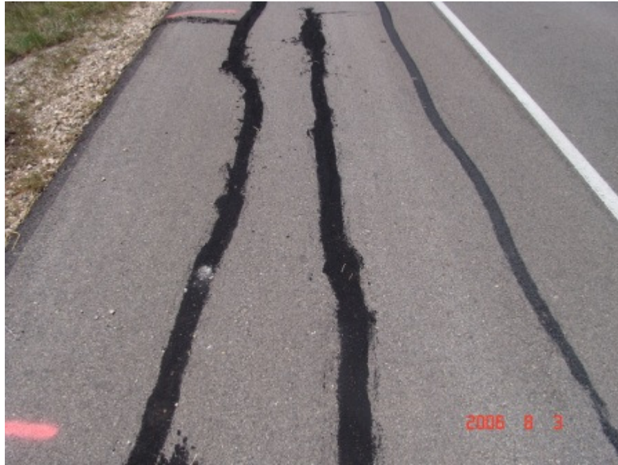
Figure A-37 Control section at Yoakum, TX on August 2006 (Part 1)
