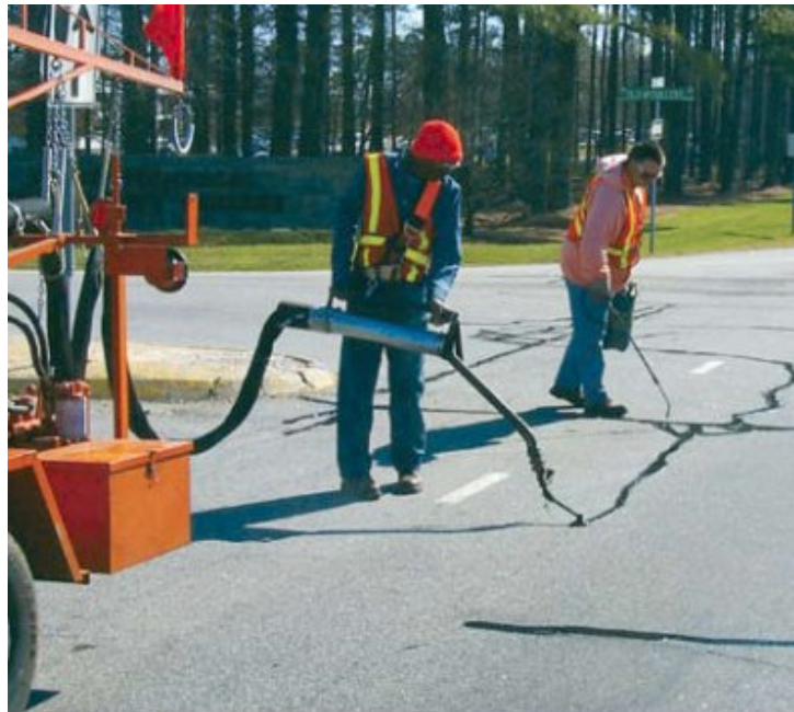
Figure 6-47 Typical crack sealing process (fhwa.dot.gov)
