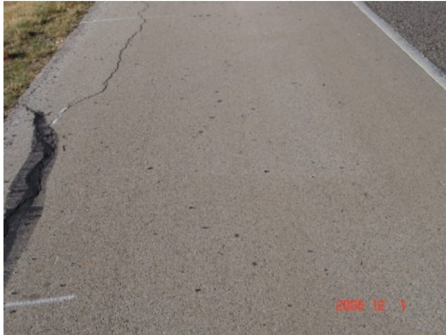
Figure A-5 DMC_1 section at Stephenville, TX on December 2006 (Part 1)
