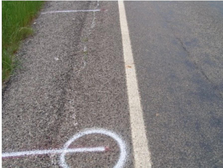
Figure A-93 Control section at Tyler, TX on April 2007 (Part 4)
