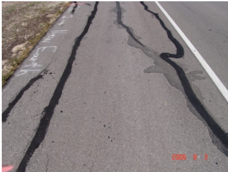
Figure A-32 WBSC_1 section at Yoakum, TX on August 2006 (Part 4)
