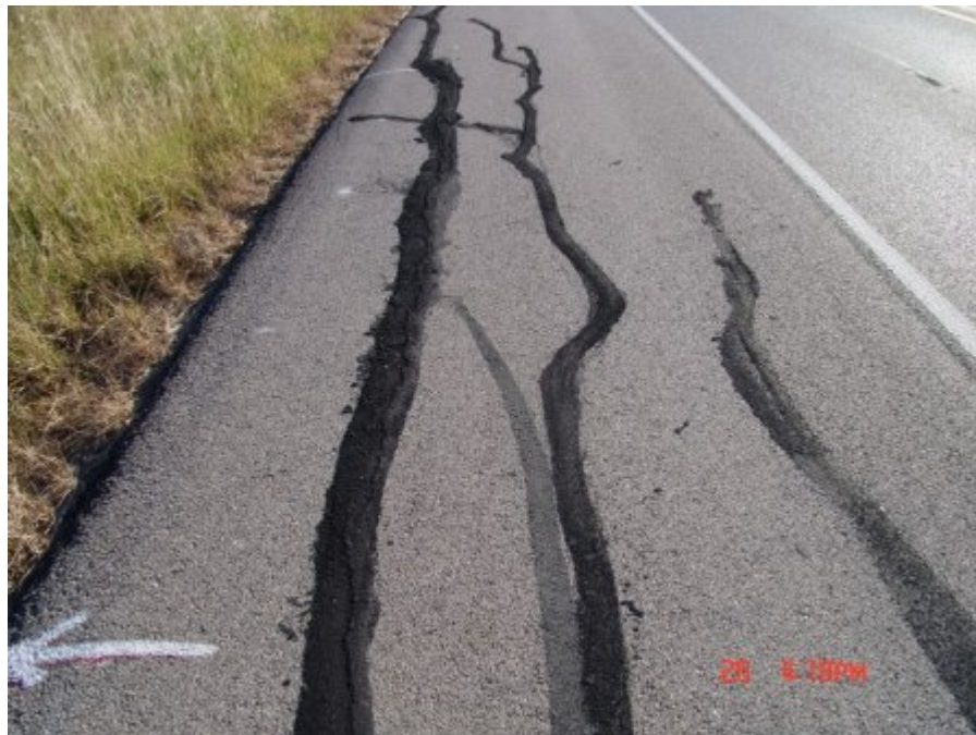
Figure A-64 Control section at Yoakum, TX on October 2007 (Part 4)
