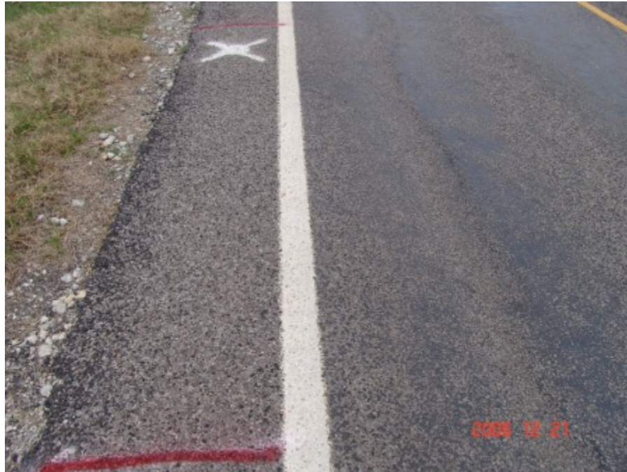
Figure A-67 Control section at Tyler, TX on December 2006 (Part 1)
