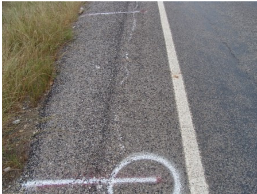
Figure A-100 Control section at Tyler, TX on May 2007 (Part 3)
