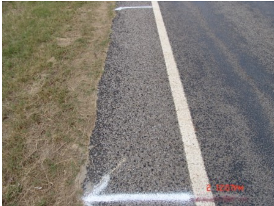
Figure A-113 Control section at Tyler, TX on October 2007 (Part 1)
