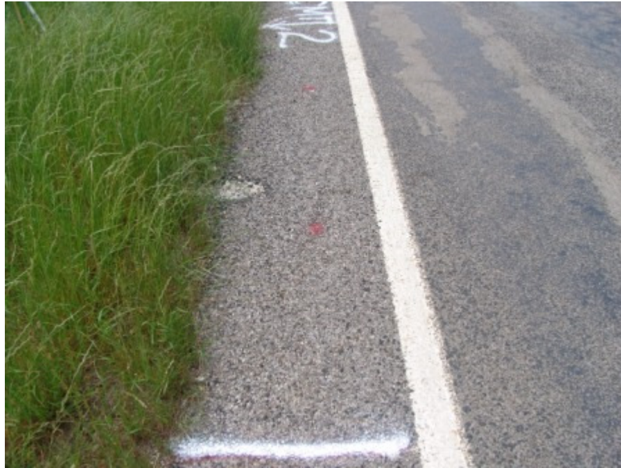
Figure A-89 WC_3 compost treated section at Tyler, TX on April 2007
