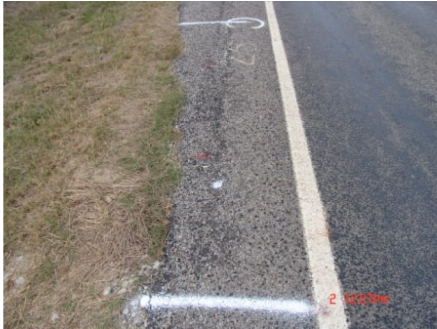
Figure A-115 Control section at Tyler, TX on October 2007 (Part 3)
