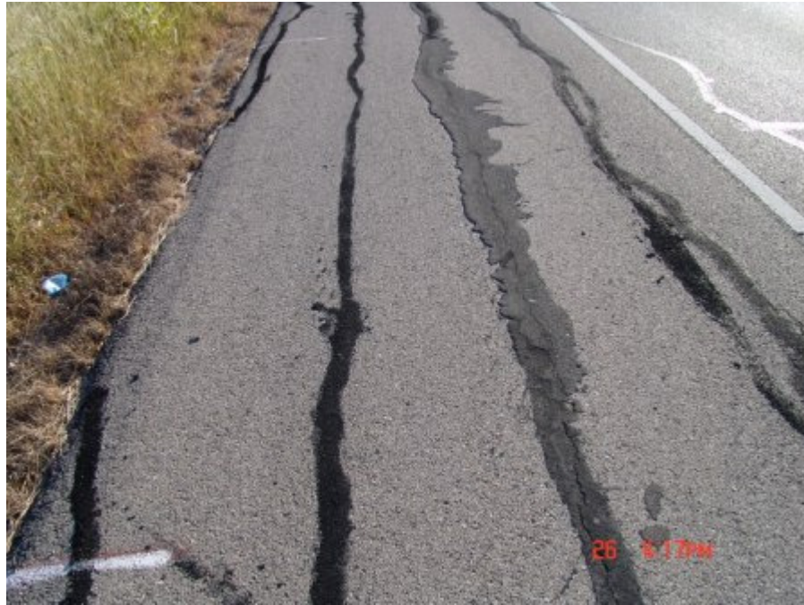
Figure A-57 WC_1 section at Yoakum, TX on October 2007 (Part 1)
