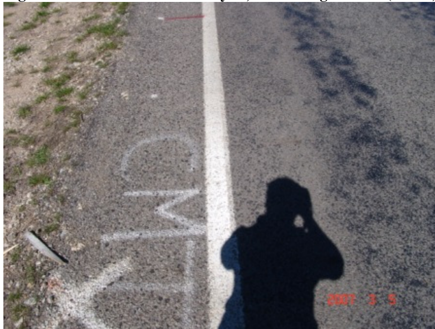
Figure A-80 WC_2 compost treated section at Tyler, TX on March 2007
