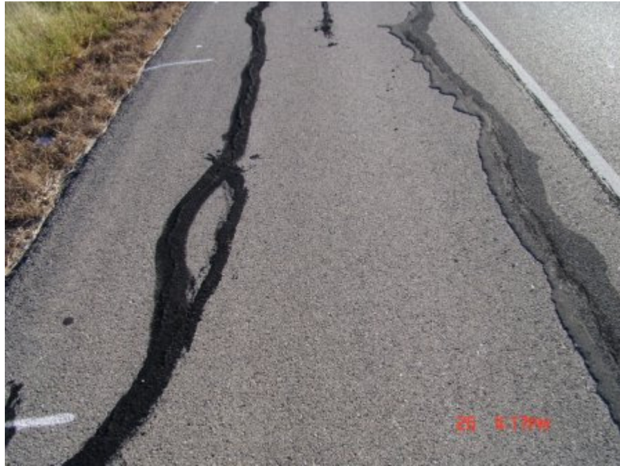
Figure A-53 WBSC_1 section at Yoakum, TX on October 2007 (Part 1)
