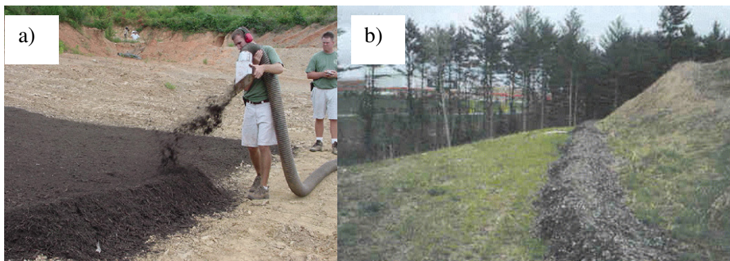
Figure 2-3 (a) Application of compost blanket, (b) Compost filter berm at the end of a steep slope
