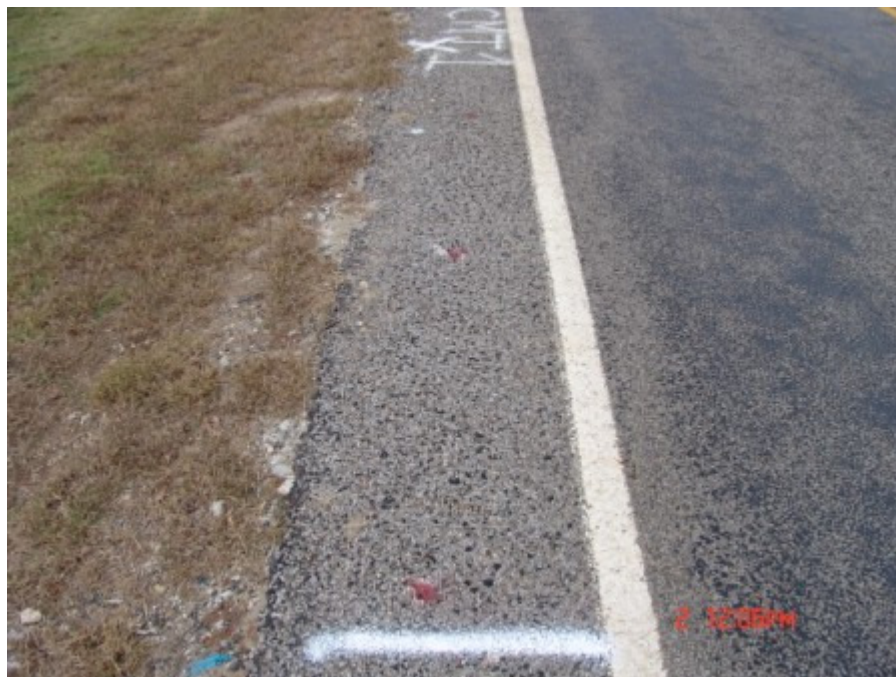
Figure A-112 WC_2 compost treated section at Tyler, TX on October 2007
