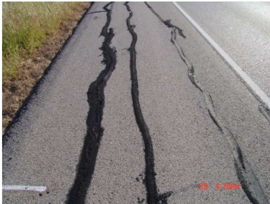
Figure A-62 Control section at Yoakum, TX on October 2007 (Part 2)
