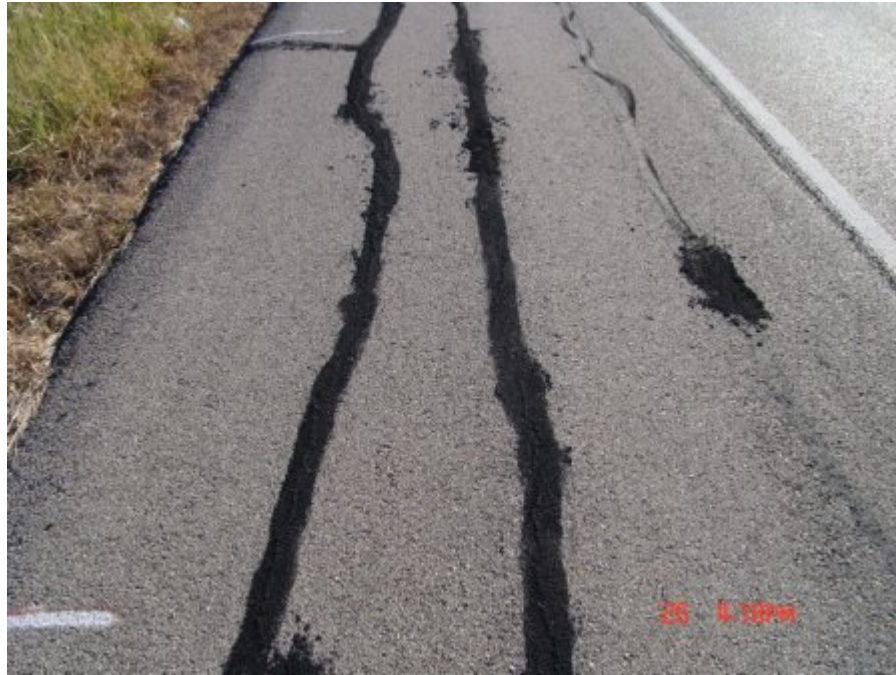
Figure A-61 Control section at Yoakum, TX on October 2007 (Part 1)
