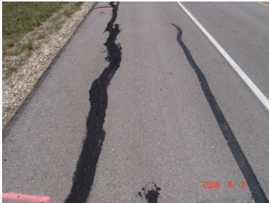
Figure A-38 Control section at Yoakum, TX on August 2006 (Part 2)
