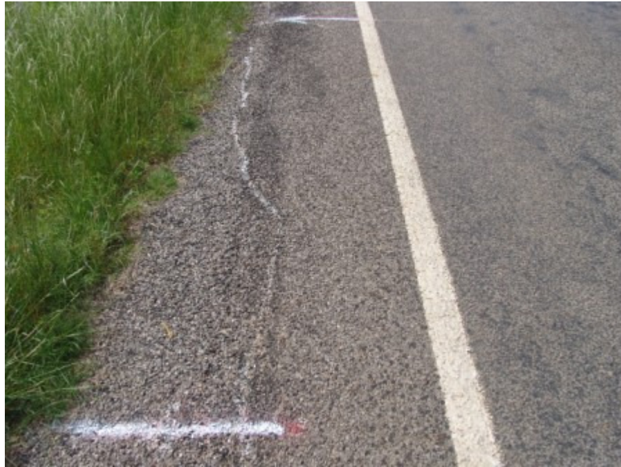
Figure A-95 Control section at Tyler, TX on April 2007 (Part 6)
