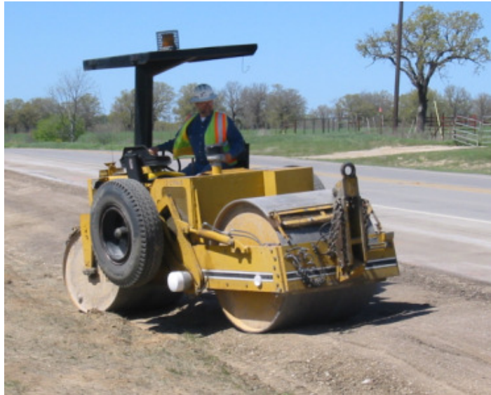
Figure 4-9 Compaction of the CMT using smooth drum roller
