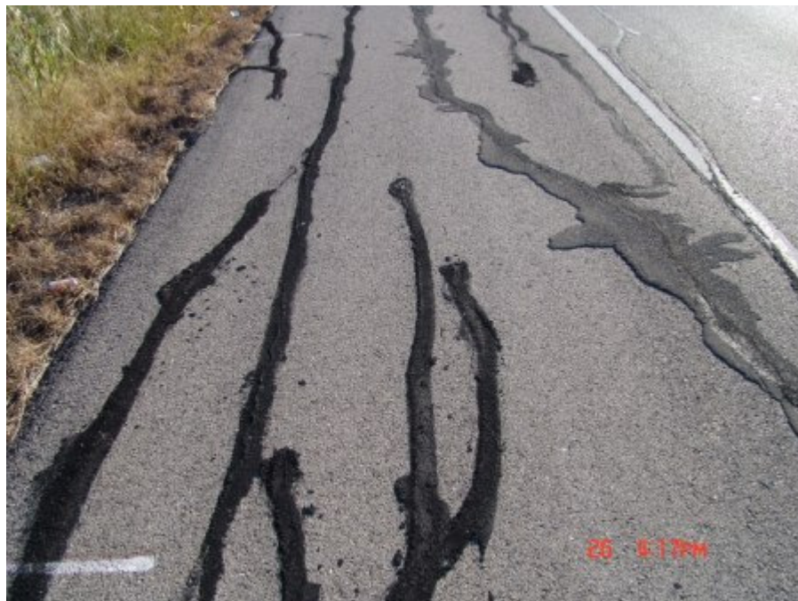
Figure A-56 WBSC_1 section at Yoakum, TX on October 2007 (Part 4)
