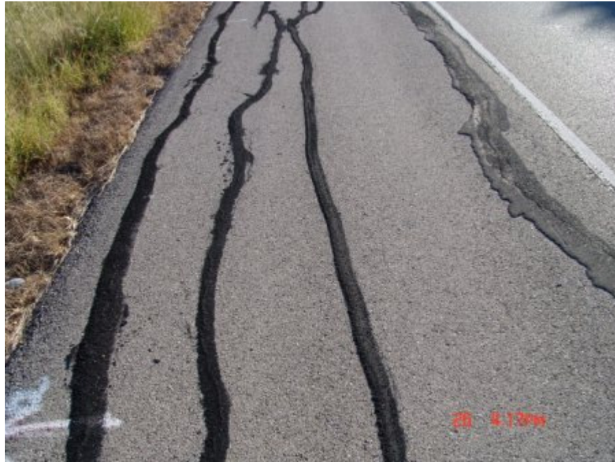
Figure A-55 WBSC_1 section at Yoakum, TX on October 2007 (Part 3)
