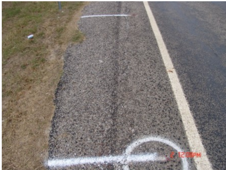
Figure A-116 Control section at Tyler, TX on October 2007 (Part 4)
