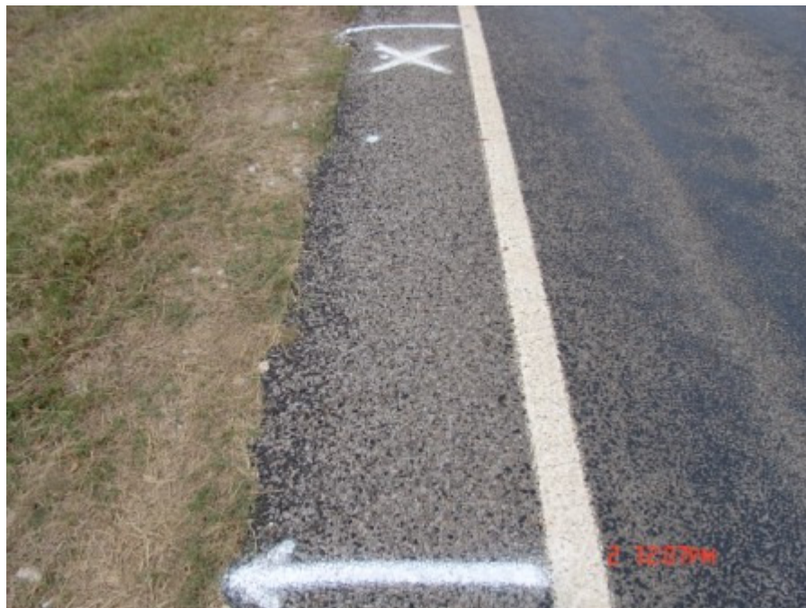
Figure A-114 Control section at Tyler, TX on October 2007 (Part 2)
