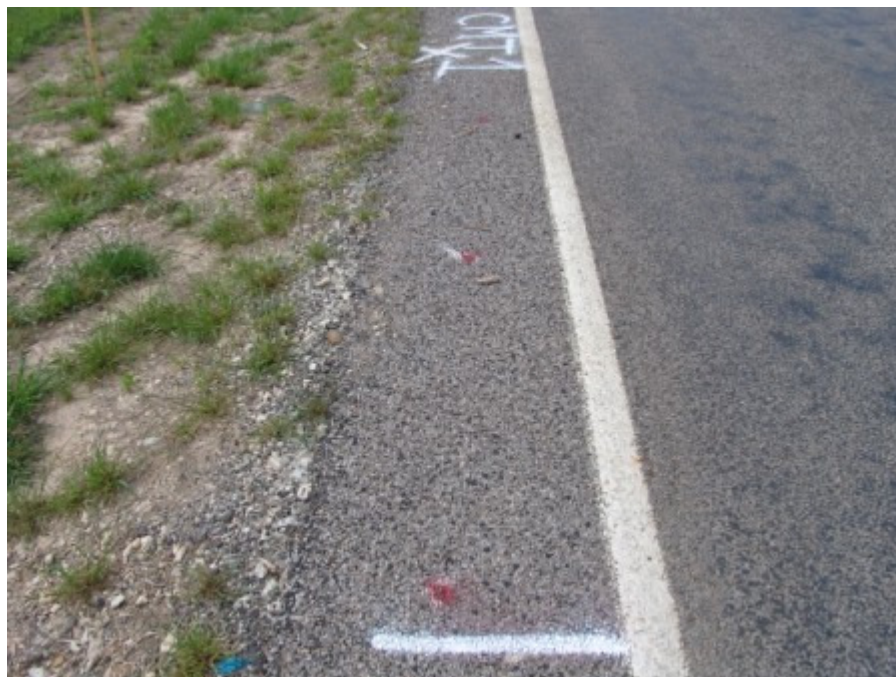
Figure A-88 WC_2 compost treated section at Tyler, TX on April 2007
