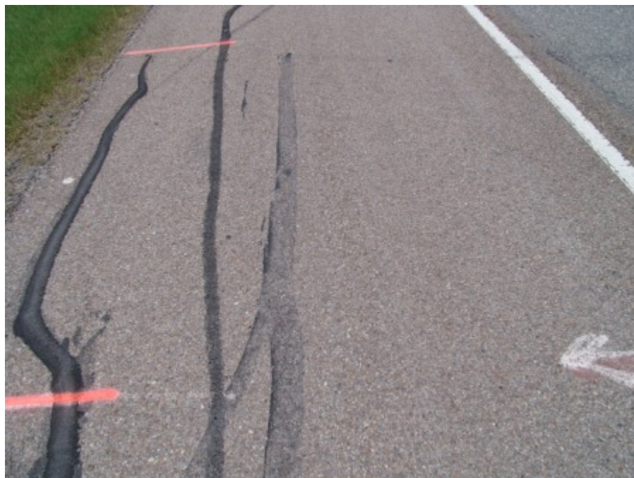
Figure A-24 Control section at Corpus Christi, TX May 2007 (Part 2)
