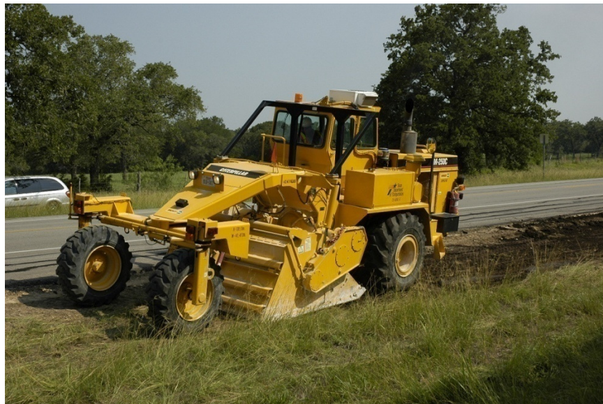
Figure 4-7 Tiller used for mixing the soil and compost
