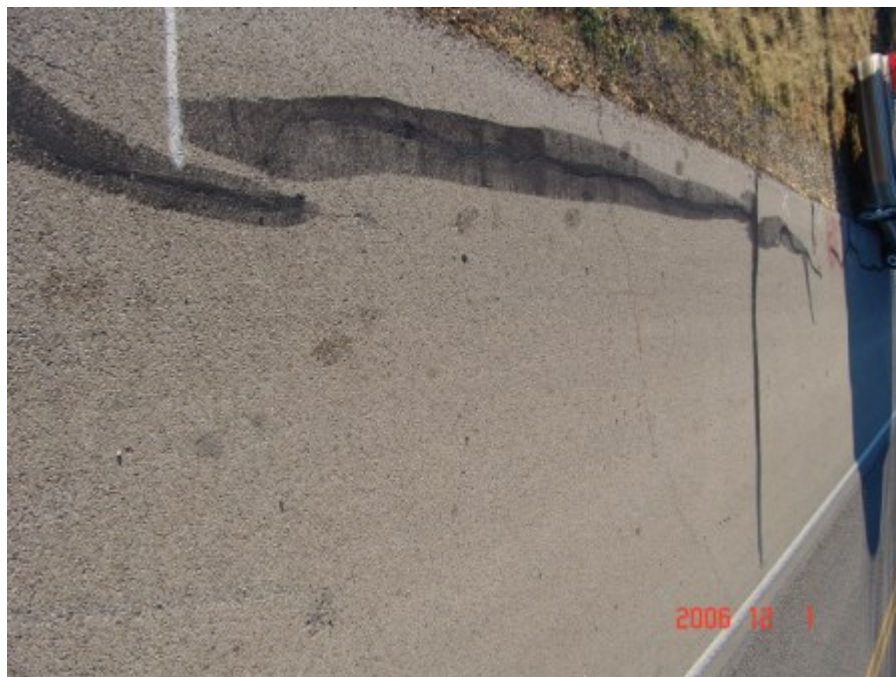
Figure A-8 Control Section at Stephenville, TX on December 2006 (Part 2)
