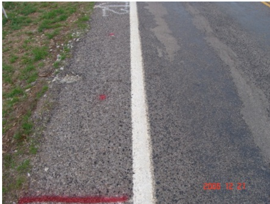
Figure A-66 WC_3 compost treated section at Tyler, TX on December 2006
