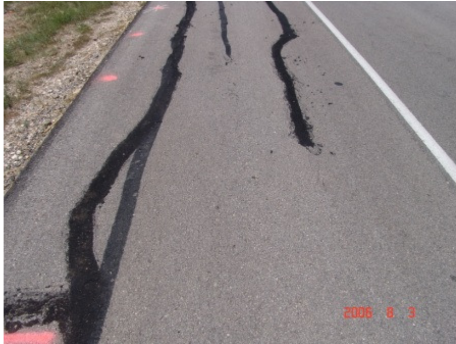
Figure A-39 Control section at Yoakum, TX on August 2006 (Part 3)
