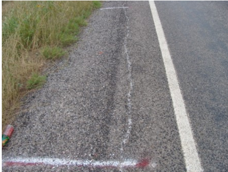
Figure A-101 Control section at Tyler, TX on May 2007 (Part 4)
