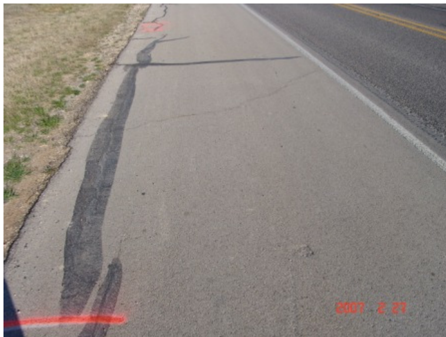
Figure A-12 Control Section at Stephenville, TX on February 2007 (part 2)
