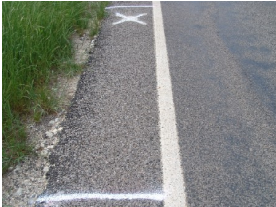
Figure A-91 Control section at Tyler, TX on April 2007 (Part 2)
