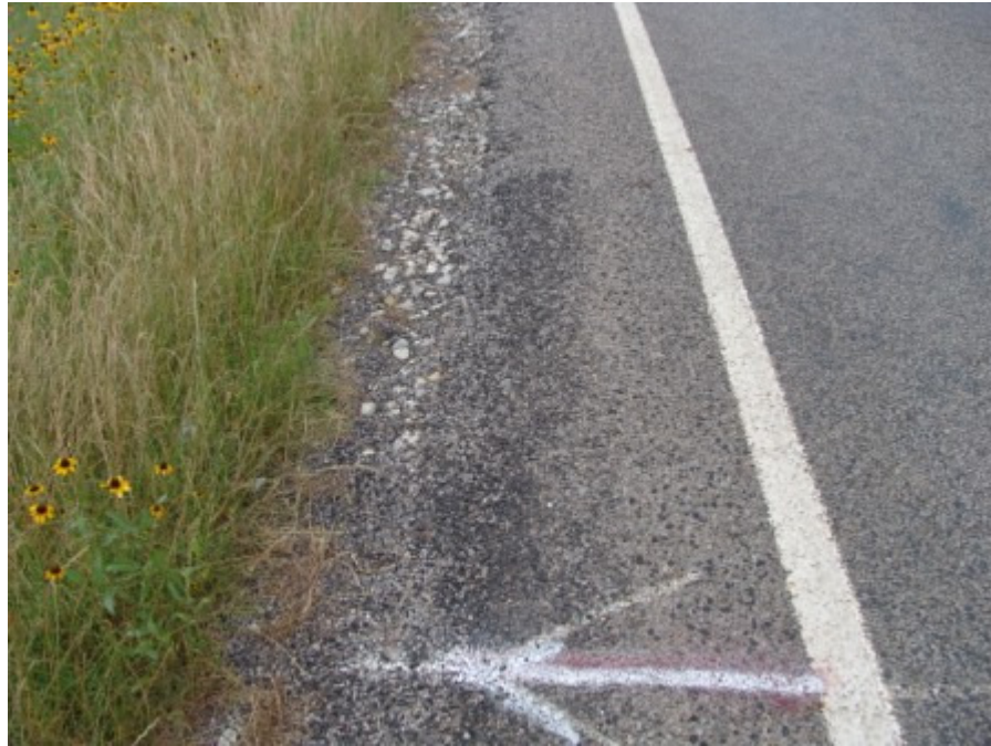
Figure A-103 Control section at Tyler, TX on May 2007 (Part 6)
