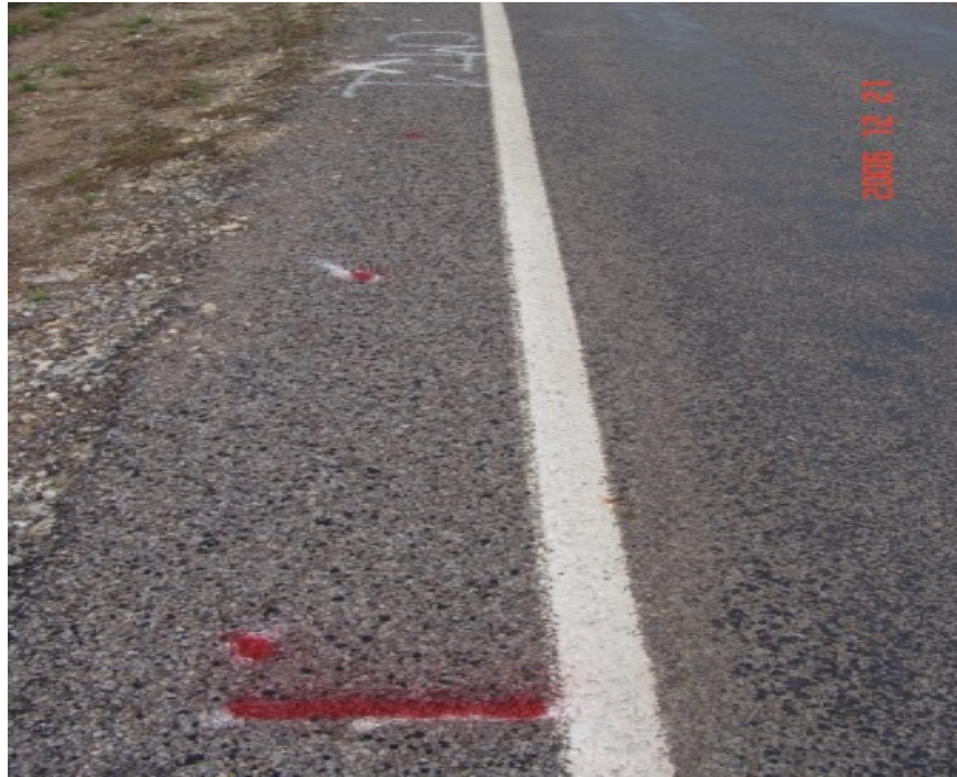
Figure A-65 WC_2 compost treated section at Tyler, TX on December 2006
