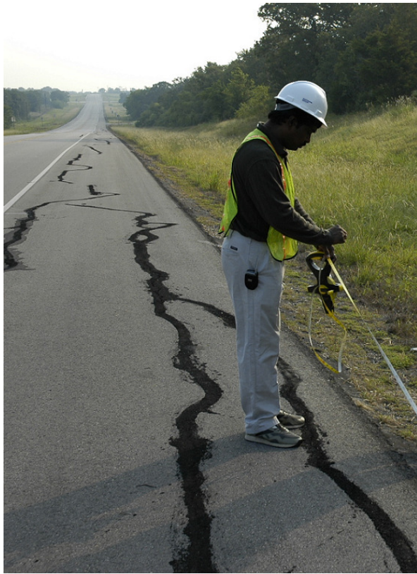
Figure 4-3 Yoakum, TX test site before field construction
