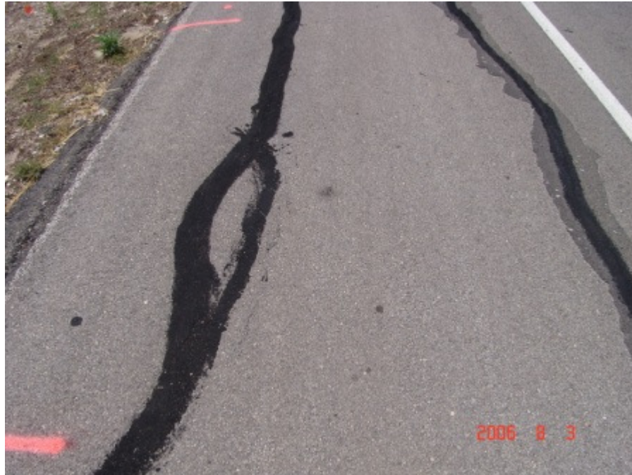
Figure A-29 WBSC_1 section at Yoakum, TX on August 2006 (Part 1)
