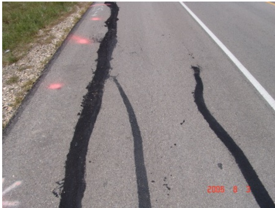
Figure A-40 Control section at Yoakum, TX on August 2006 (Part 4)
