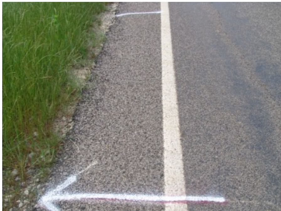
Figure A-90 Control section at Tyler, TX on April 2007 (Part 1)
