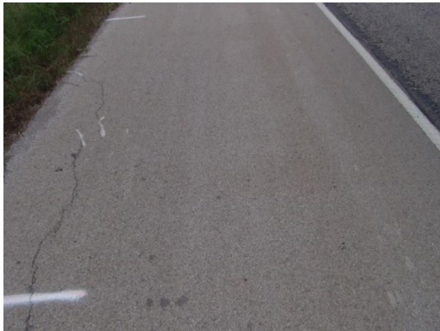
Figure A-14 DMC_1 section at Stephenville, TX on December 2007 (Part 2)
