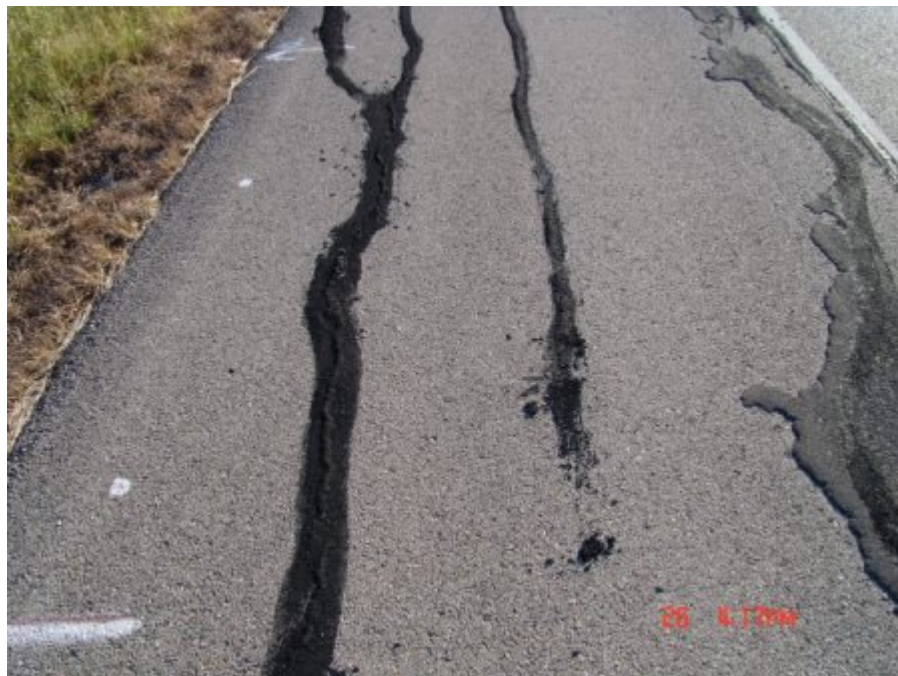
Figure A-54 WBSC_1 section at Yoakum, TX on October 2007 (Part 2)
