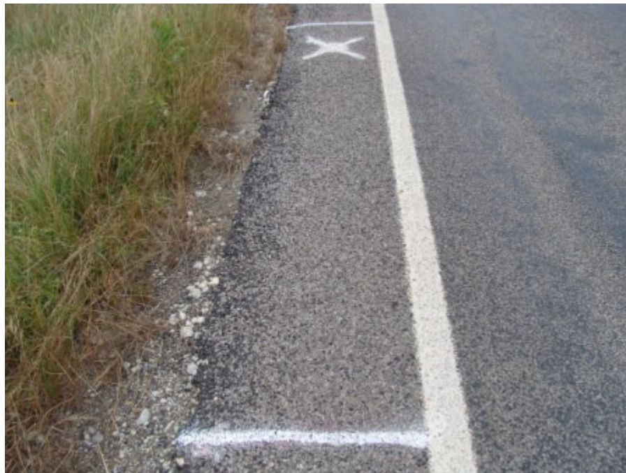
Figure A-98 Control section at Tyler, TX on May 2007 (Part 1)
