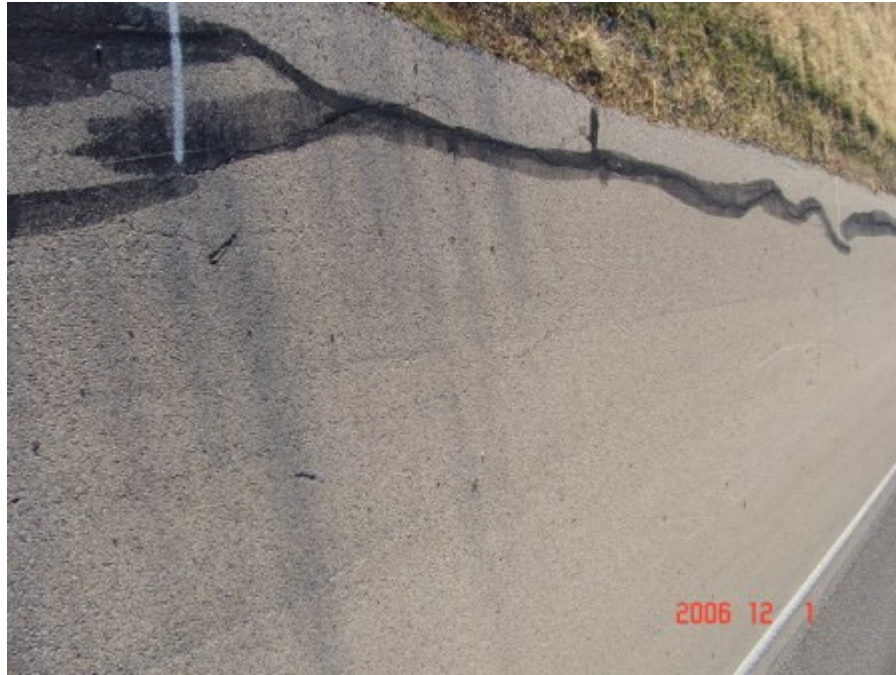
Figure A-7 Control Section at Stephenville, TX on December 2006 (Part 1)
