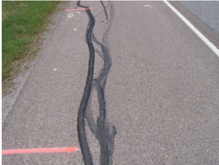
Figure A-23 Control section at Corpus Christi, TX May 2007 (Part 1)
