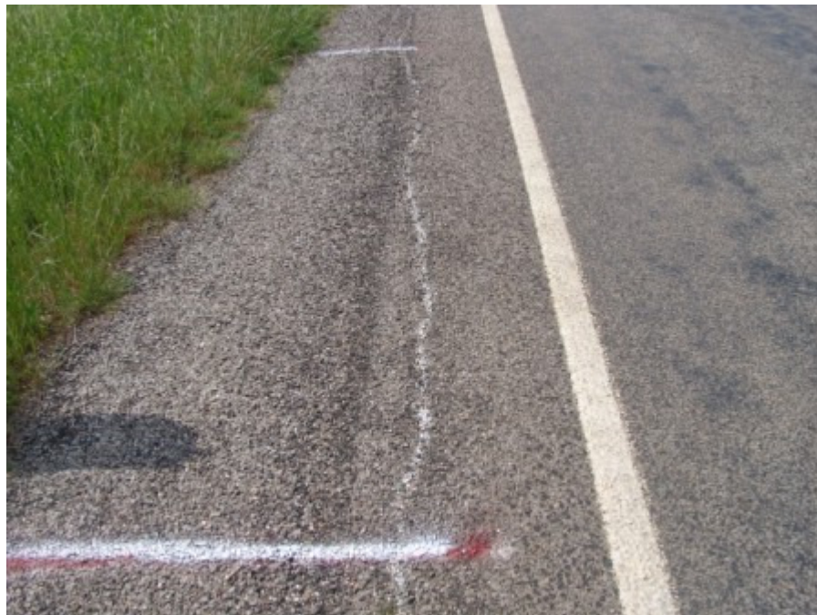
Figure A-94 Control section at Tyler, TX on April 2007 (Part 5)
