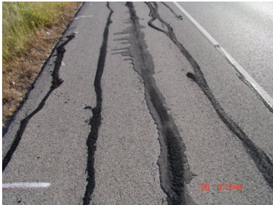
Figure A-58 WC_1 section at Yoakum, TX on October 2007 (Part 2)
