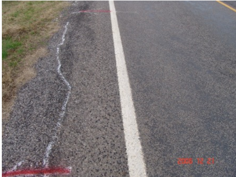
Figure A-71 Control section at Tyler, TX on December 2006 (Part 5)
