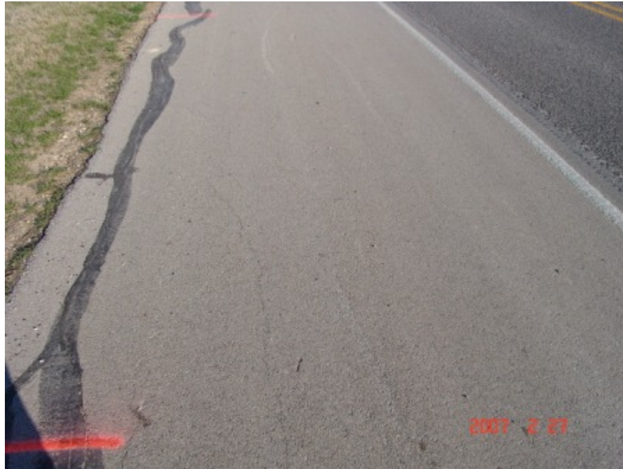
Figure A-11 Control Section at Stephenville, TX on February 2007 (part 1)
