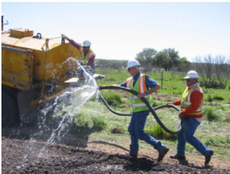
Figure 4-8 Application of water onto the CMT
