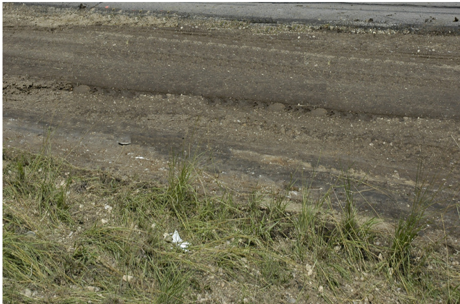
Figure 4-10 Completed CMT section
