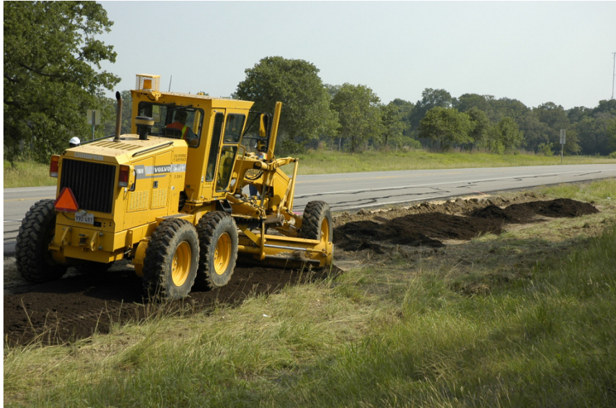
Figure 4-6 Application of a compost layer over the tilled site soil
