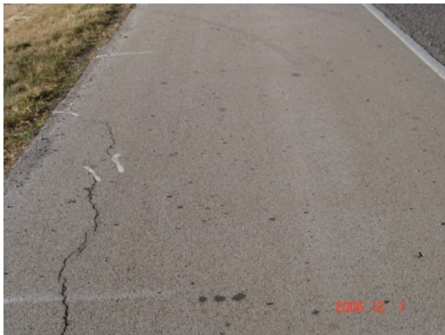
Figure A-6 DMC_1 section at Stephenville, TX on December 2006 (Part 2)
