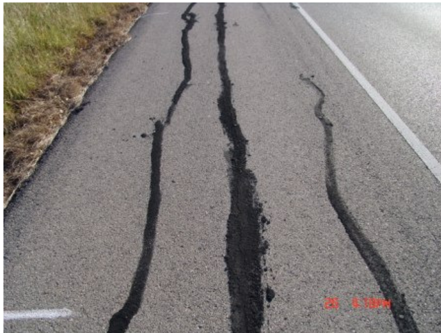
Figure A-60 WC_1 section at Yoakum, TX on October 2007 (Part 4)
