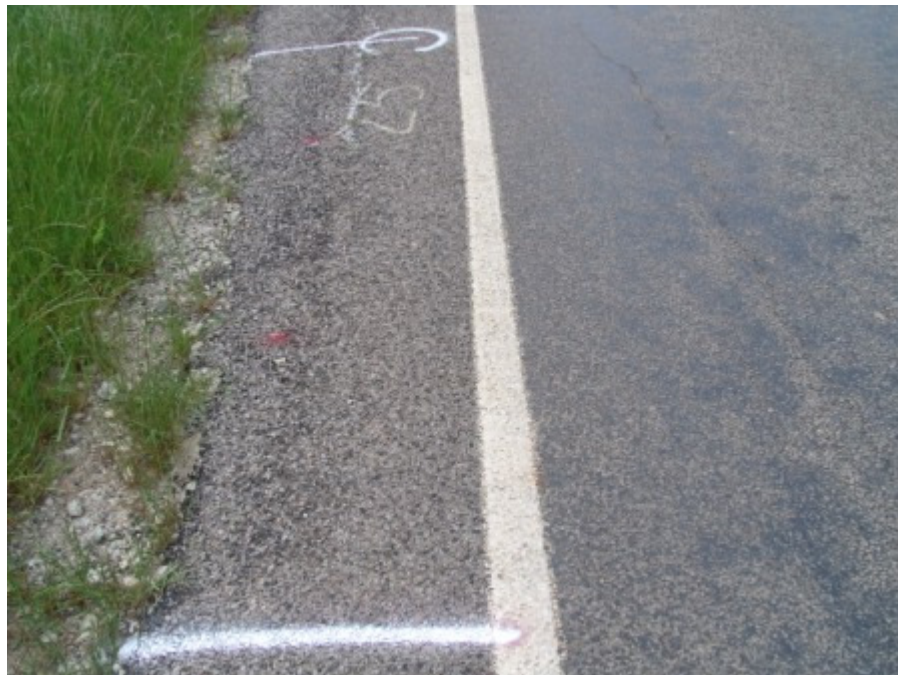
Figure A-92 Control section at Tyler, TX on April 2007 (Part 3)
