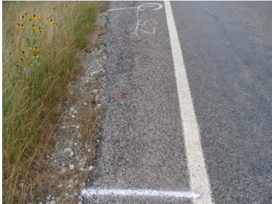
Figure A-99 Control section at Tyler, TX on May 2007 (Part 2)
