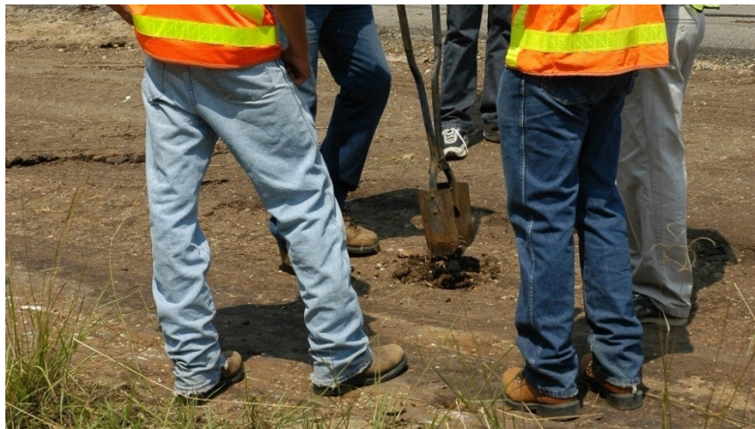
Figure 4-11 Digging holes for the moisture and temperature logger
