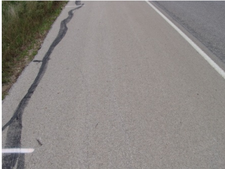
Figure A-15 Control Section at Stephenville, TX on December 2007 (part 1)
