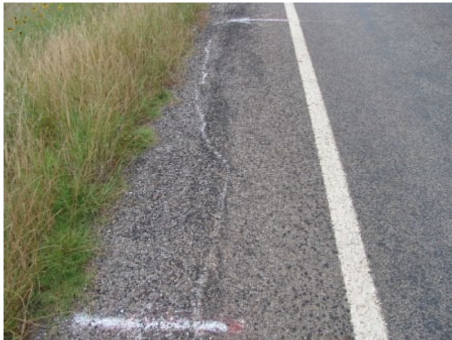
Figure A-102 Control section at Tyler, TX on May 2007 (Part 5)
