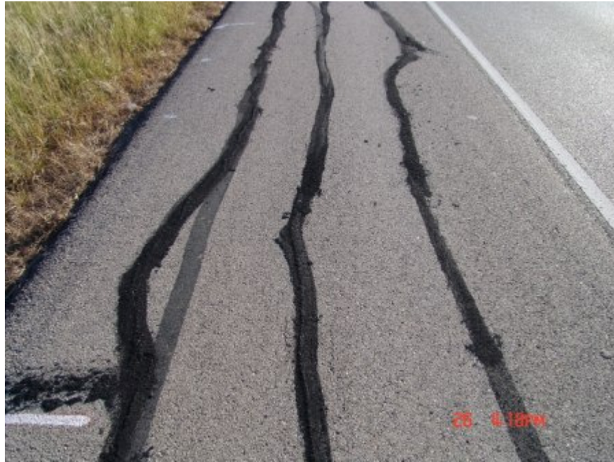
Figure A-63 Control section at Yoakum, TX on October 2007 (Part 3)
