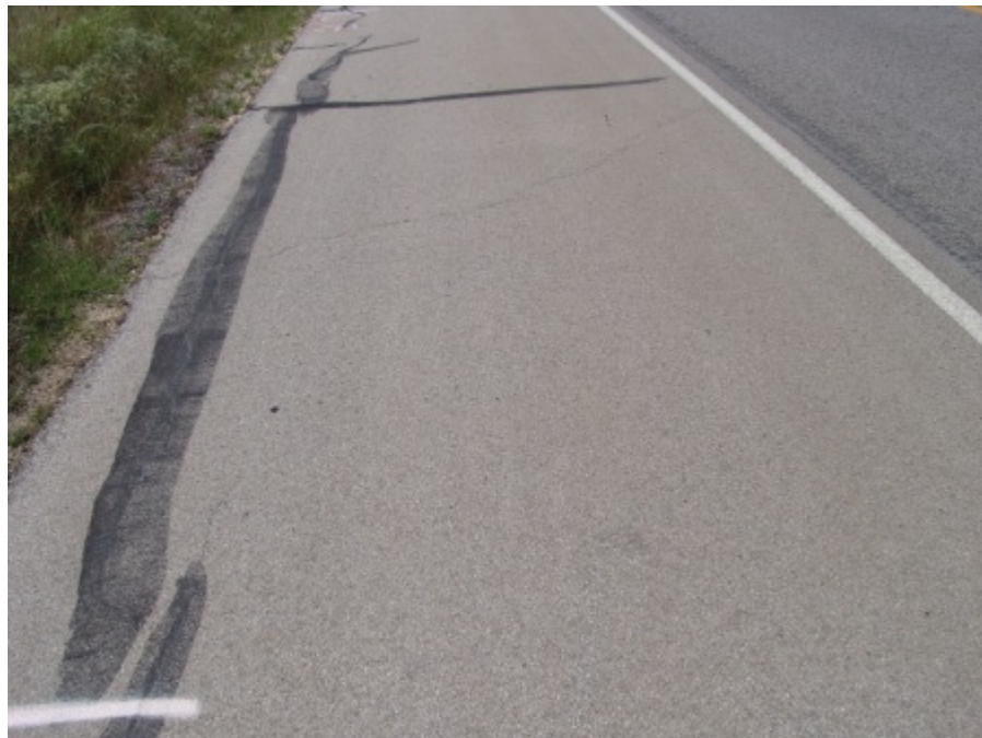
Figure A-16 Control Section at Stephenville, TX on December 2007 (part 2)
