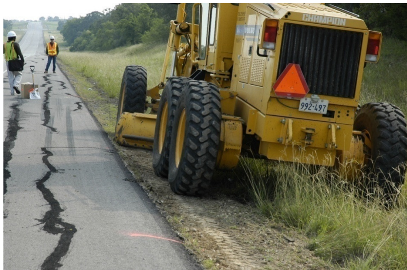
Figure 4-4 Grader used for scarifying top soil layer
