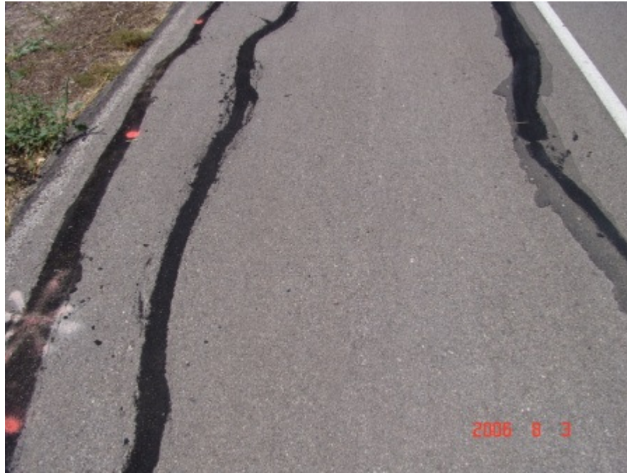
Figure A-31 WBSC_1 section at Yoakum, TX on August 2006 (Part 3)
