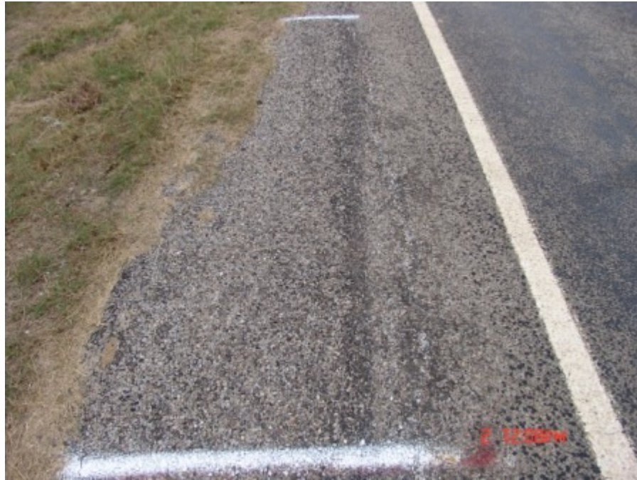
Figure A-117 Control section at Tyler, TX on October 2007 (Part 5)
