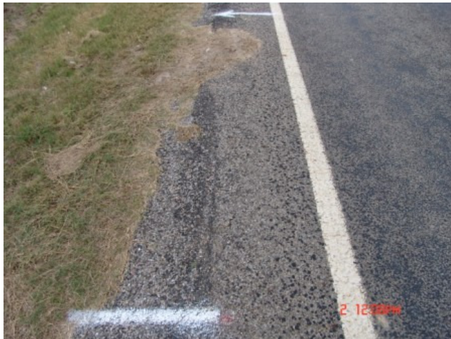
Figure A-118 Control section at Tyler, TX on October 2007 (Part 6)
