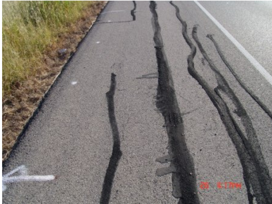
Figure A-59 WC_1 section at Yoakum, TX on October 2007 (Part 3)
