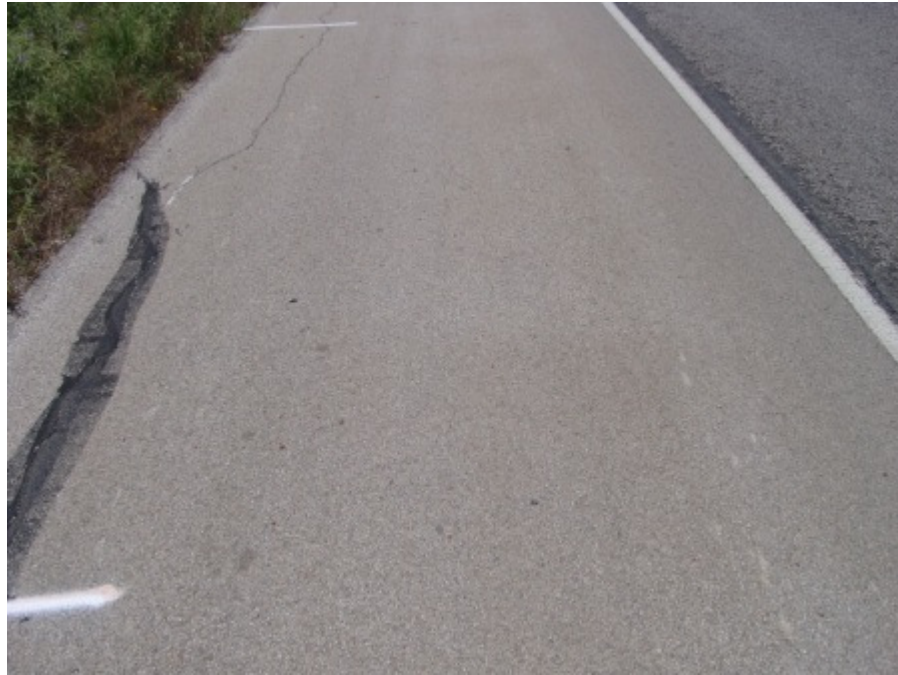
Figure A-13 DMC_1 section at Stephenville, TX on December 2007 (Part 1)
