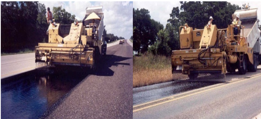
Figure 6-48 Typical application of seal coat (TTI, TAMU)
