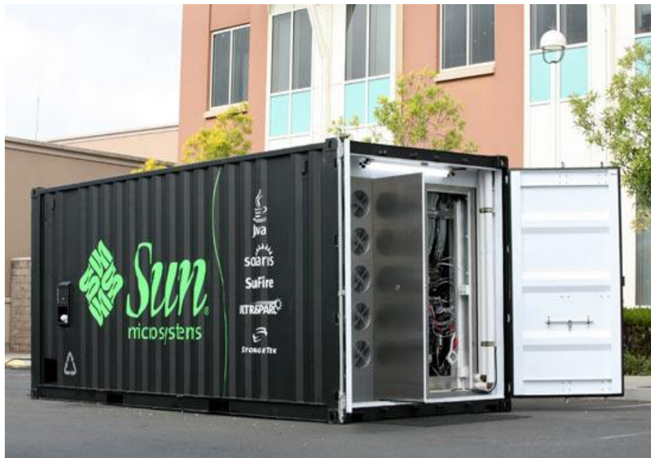
Figure 1.1: Sun Microsystems Modular Datacenter: Project Black box [3]
