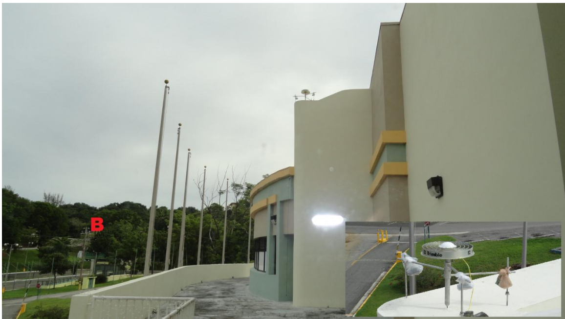
Figure A7. Photographs of site LAJ1 acquired during May 2011 campaign (A) Photoview of the antenna facing north. (B) Photoview facing east of the gymnasium building with the antenna right on top. Inset photo shows close up of antenna setup (must use a 0.5m spike mount at this site).
