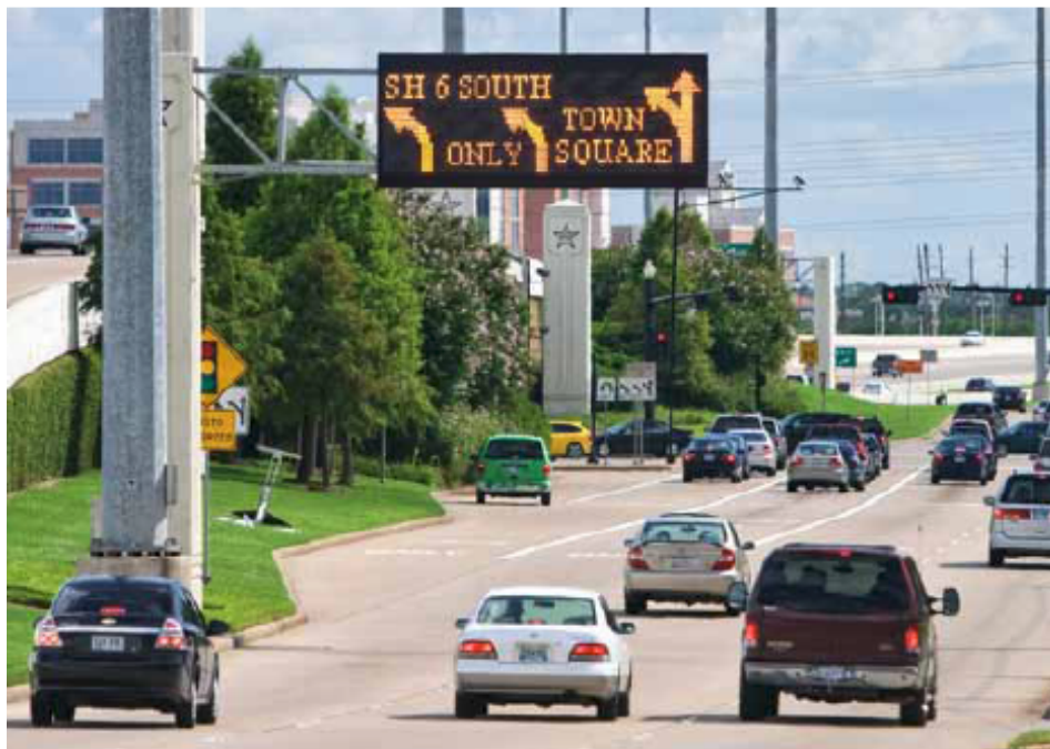
Figure 2.3 Triple Left Dynamic Message Sign, Sugar Land, Texas 13
