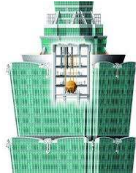
Figure 4.4 Vibration absorber at Taipei 101 (photo courtesy theengineer.co.uk).
