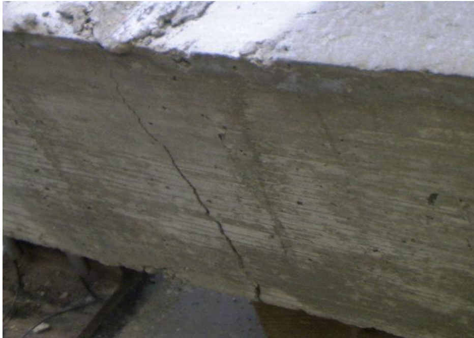
Figure 8.31: Experimental Results for the TDA concrete (7.5%TDA) Beam showing crack running at an angle to the direction of loading
