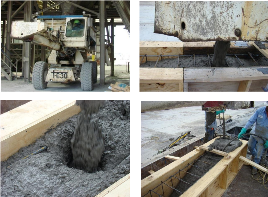
Figure 3.11 Example of Casting of Concrete Beam Specimens in the First Phase
