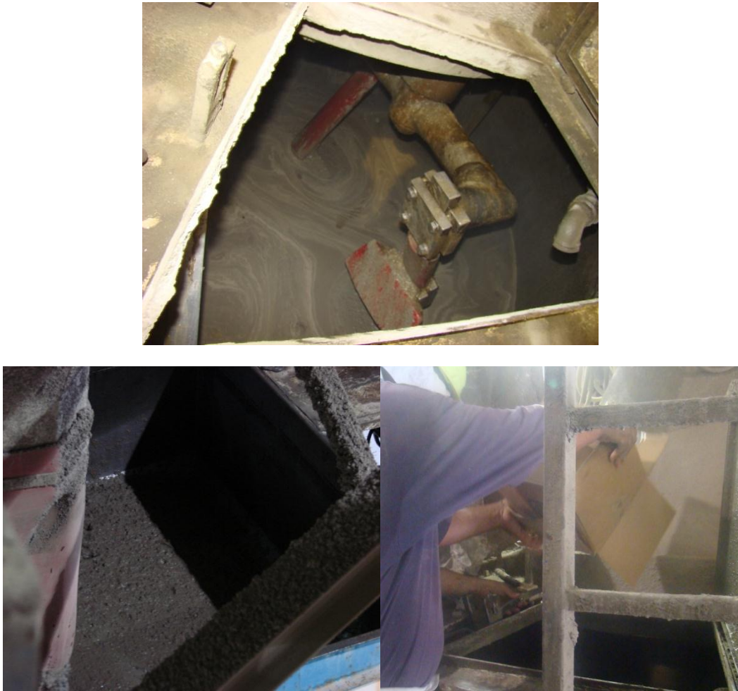
Figure 3.5 Typical Photos of Concrete Mixing
