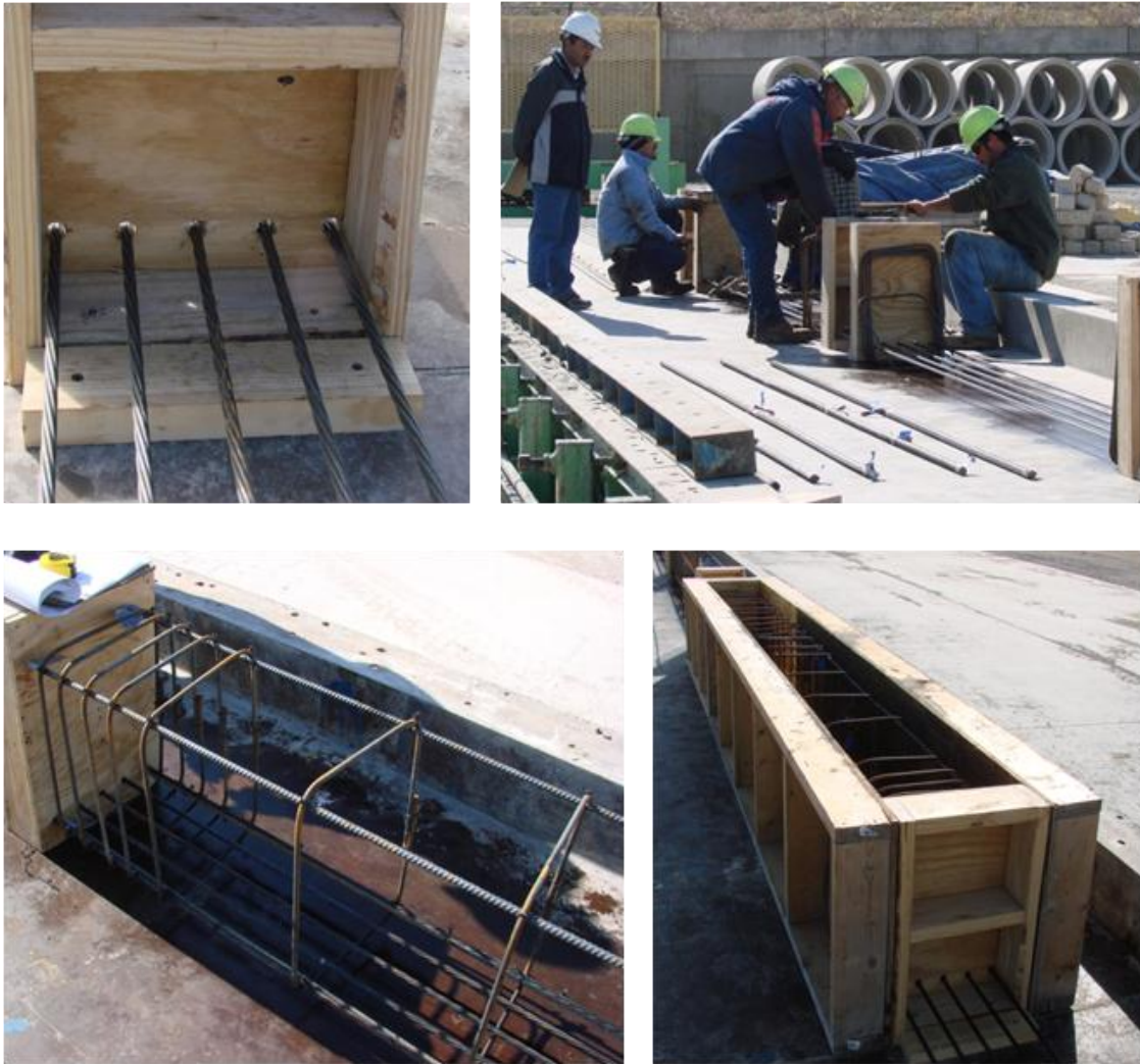
Figure 3.10 Example of Preparing Reinforcing Cages and Formworks
