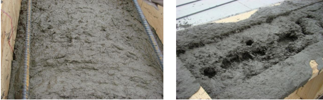
Figure 3.12 Examples of Uniformly Distributed Steel Fibers in Fresh Concrete
