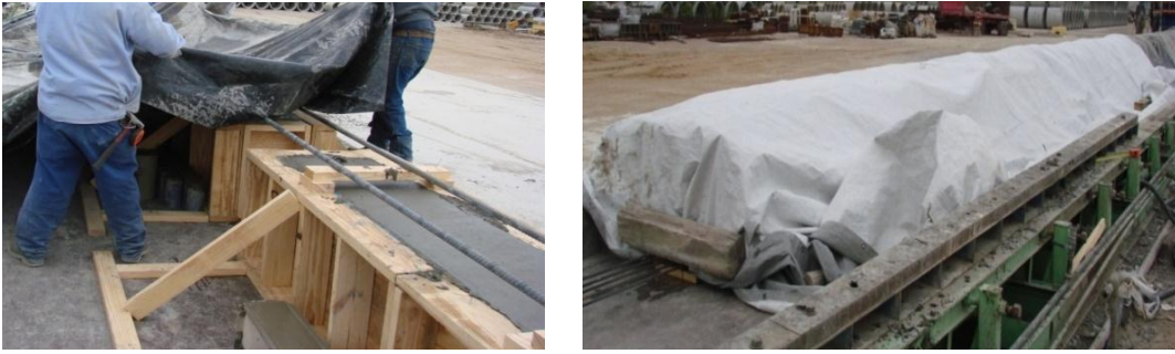
Figure 3.14 Casted Beam Covered with Plastic Sheets
