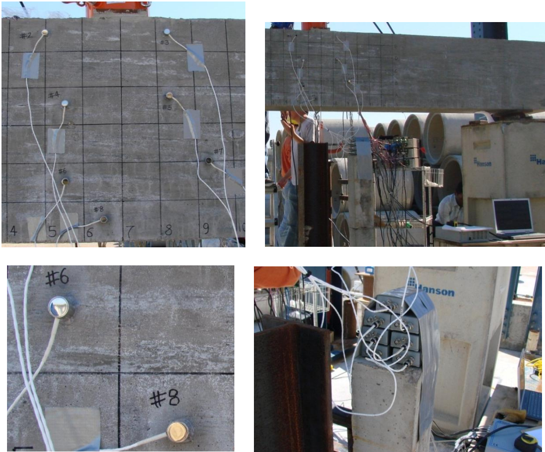
Figure 3.20 Installation of Acoustic Emission Equipments
