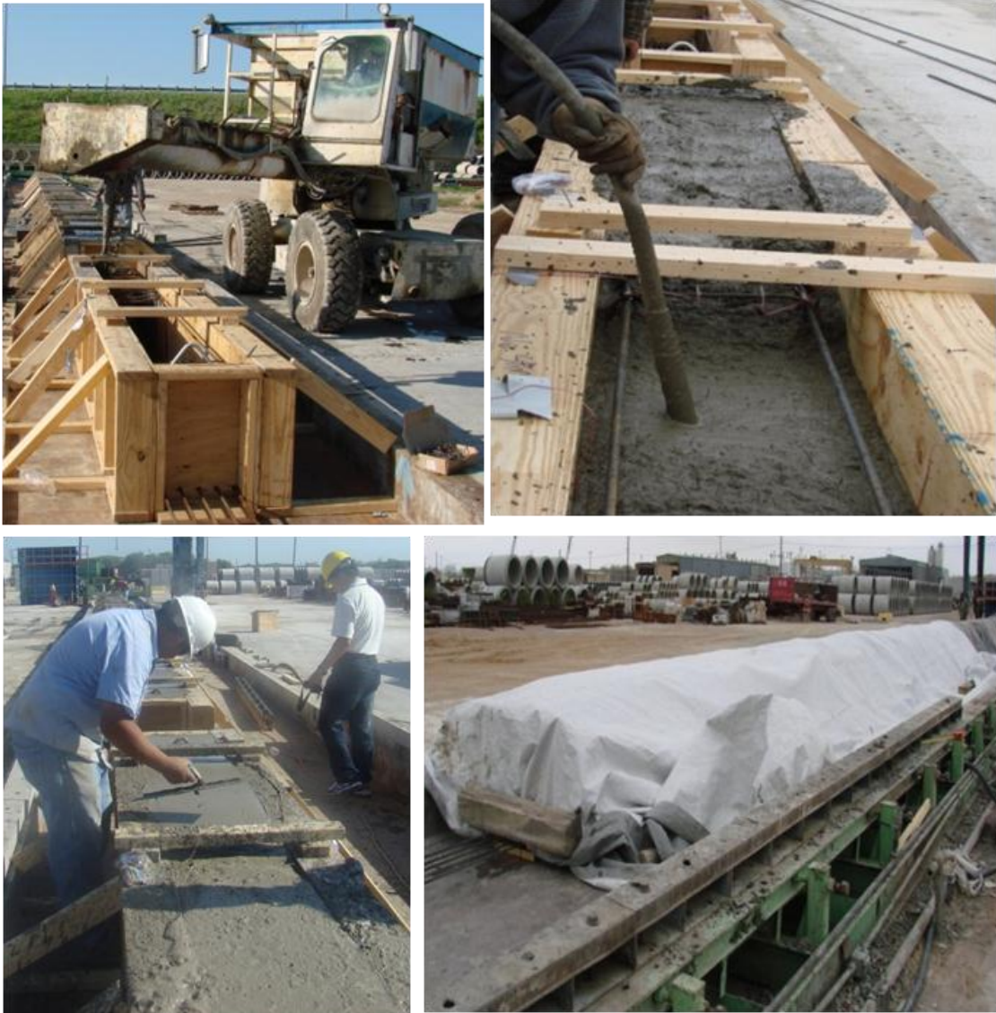
Figure 3.29 Typical Photos of Casting in Second Phase
