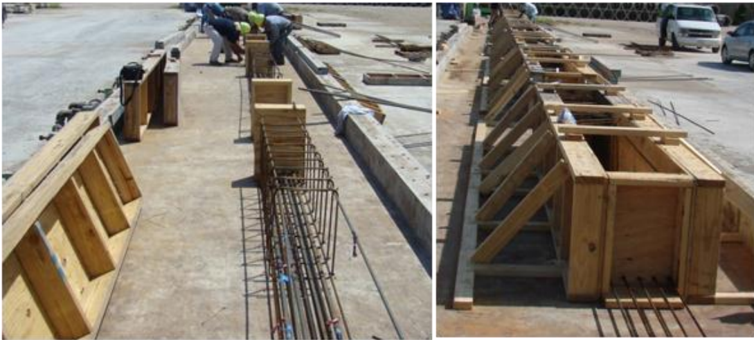
Figure 3.28 Typical Photos of Reinforcement Caging and Formworks in Second Phase
