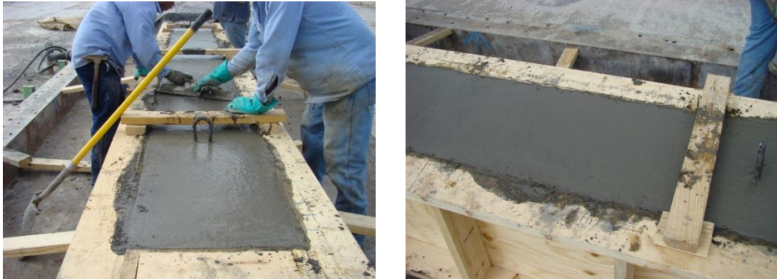
Figure 3.13 Finishing Surface after Pouring and Compacting the Fresh Concrete
