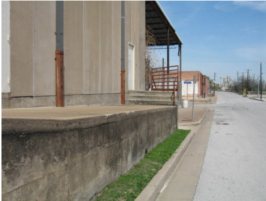
Figure 4.27 A Gap Located in the Industrial Environment (Block 44)
