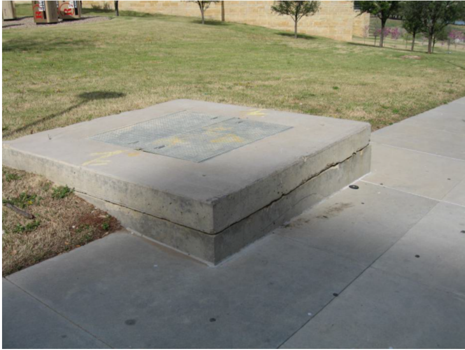
Figure 4.18 Utility Box Used by Skateboarders in a Commercial Environment (Block 1)
