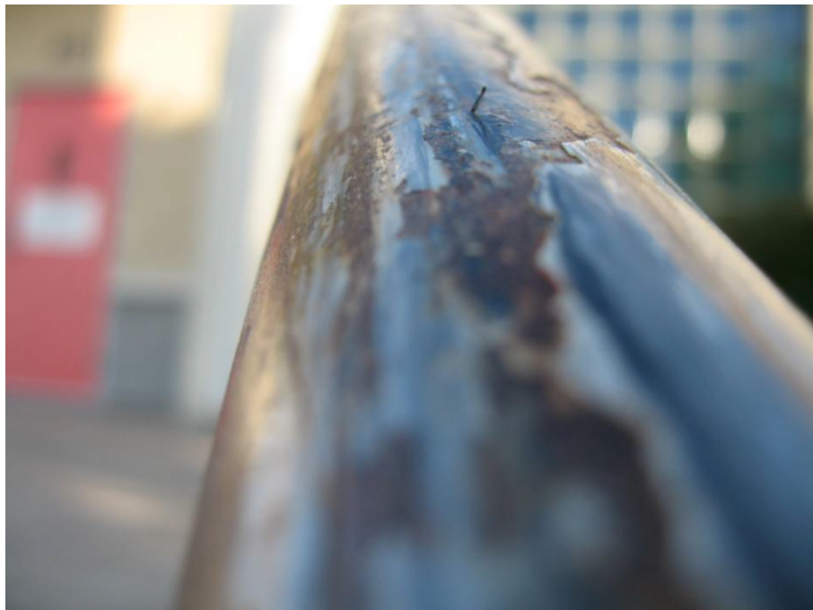
Figure 4.23 Detail of Skated Handrail (Block 37)
