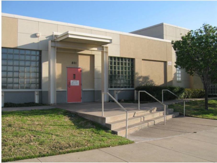
Figure 4.22 Stairs and Handrails in Educational Environment (Block 37)
