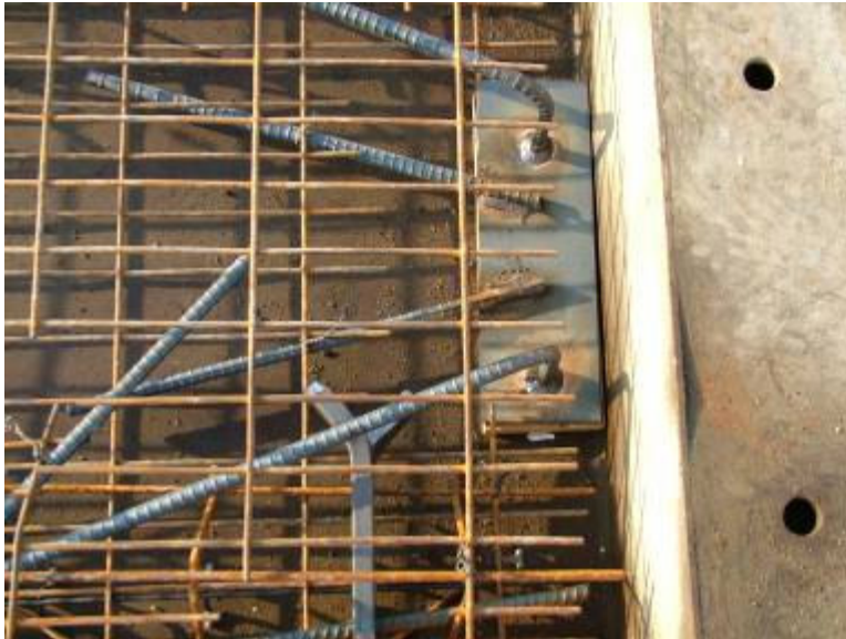
Figure A.5 Reinforcement at 45 degrees
