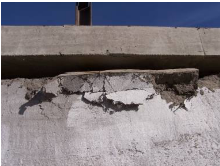
Figure D.13 Upper Middle Section of West Wall
