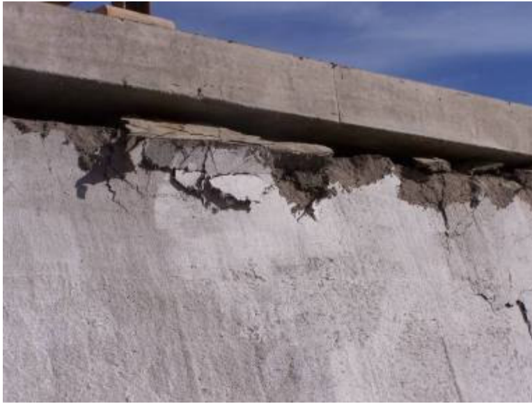
Figure D.8 Roof-West Wall View
