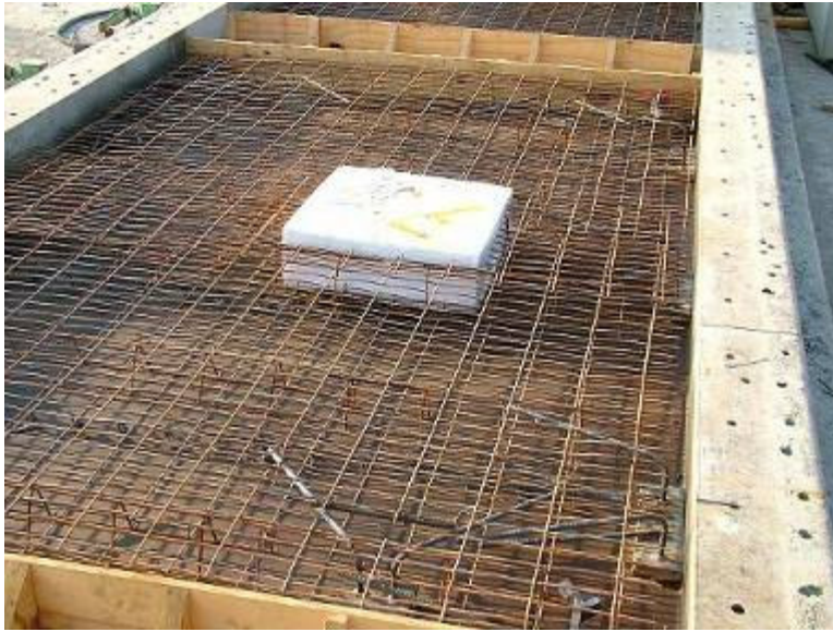
Figure A.7 Formwork for Door Panel
