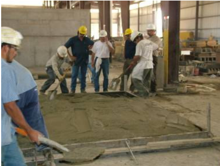
Figure A.11 Casting of Panels
