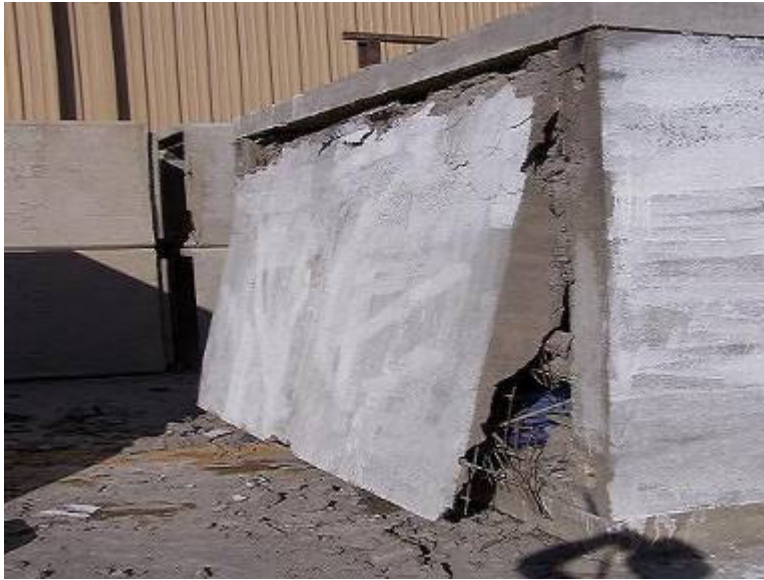
Figure D.10 West Wall
