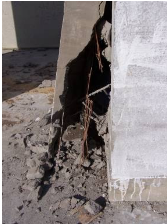
Figure D.9 Lower Right Corner of West Wall View
