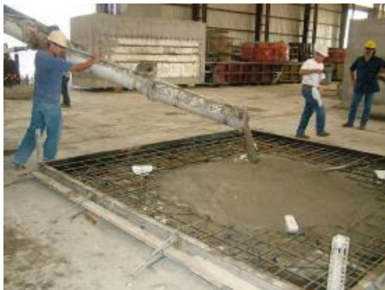
Figure 2.6 Pouring of Concrete Mix
