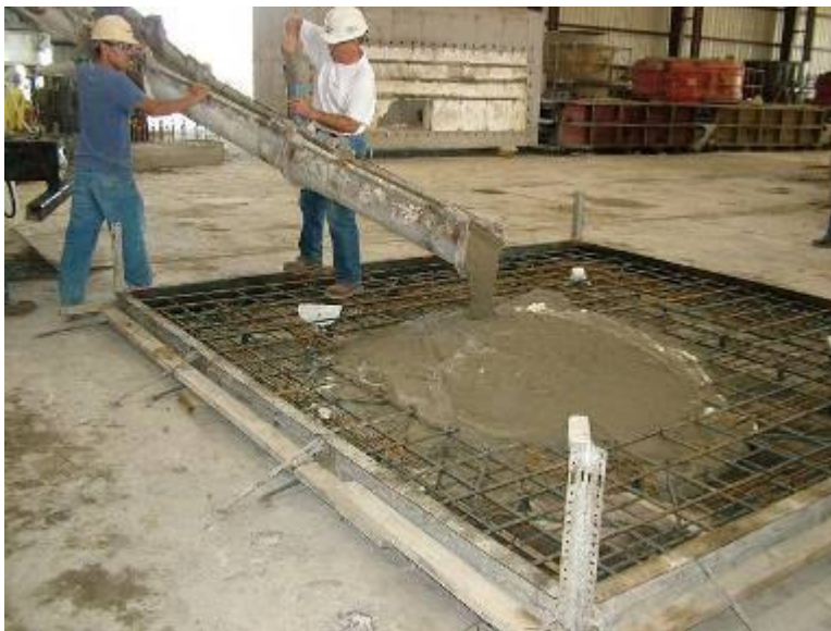
Figure A.10 Pouring of Concrete
