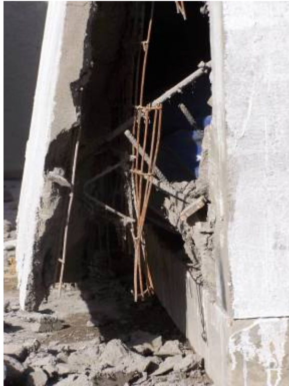
Figure D.6 Reinforcement of Panel
