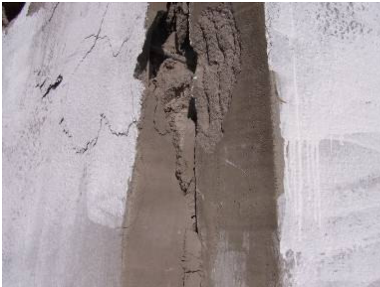
Figure D.11 Upper Right Corner View of West Wall
