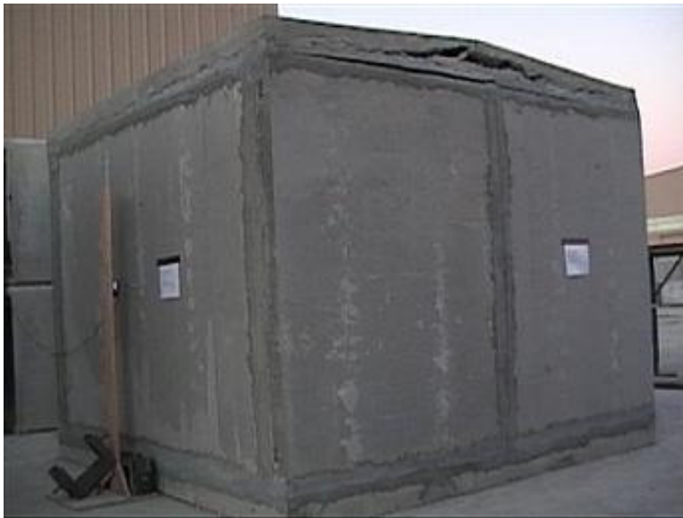
Figure C.2 Failure at Roof
