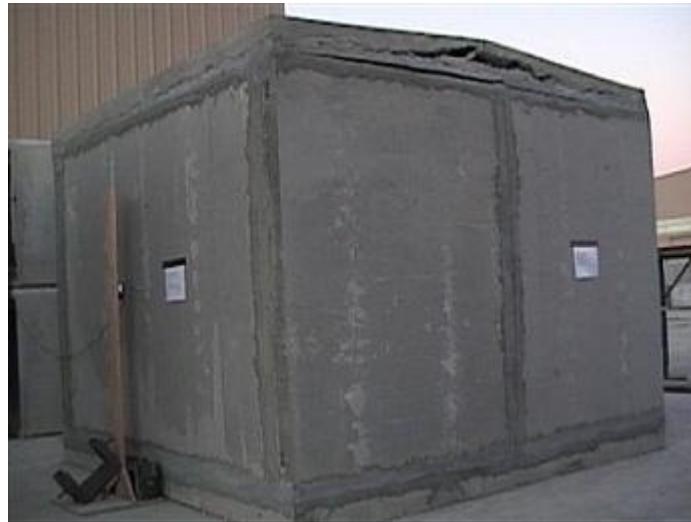
Figure 4.9 Building Prototype After Test No. 2
