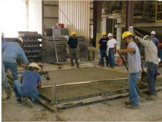
Figure 2.7 Casting of Panels
