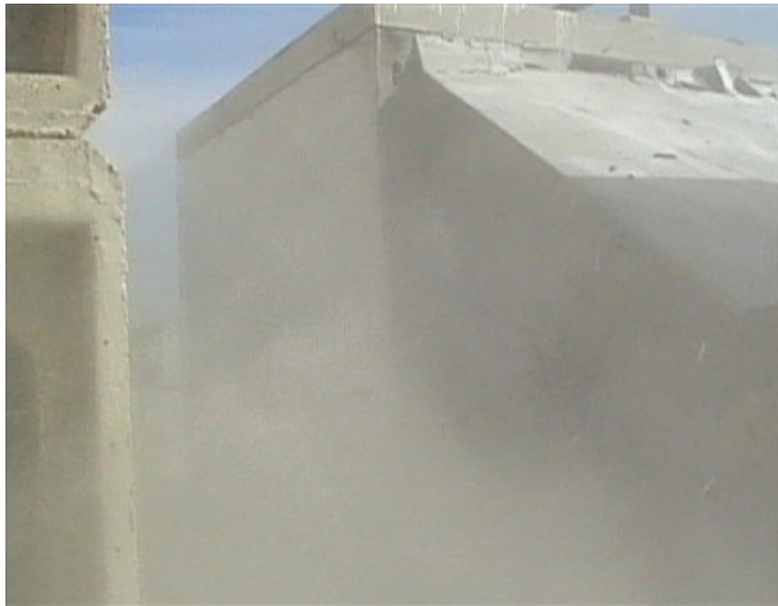
Figure 4.17 Failure of Wall Sequence 5
