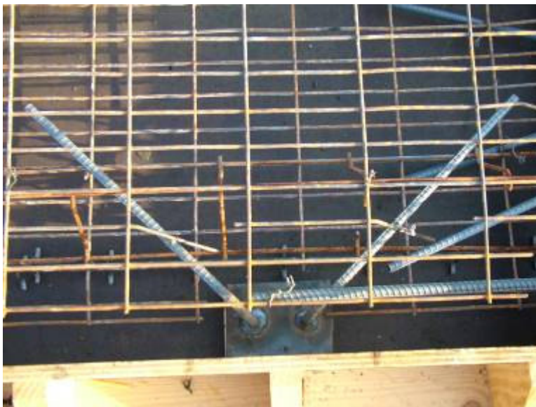
Figure A.6 Reinforcement at 45 degrees
