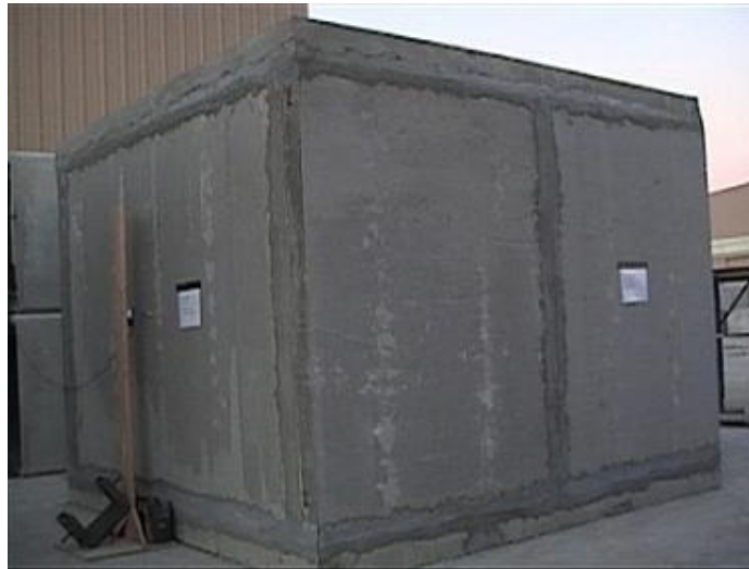
Figure 4.8 Building Prototype Before Test No. 2
