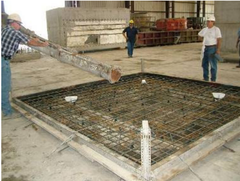
Figure A.9 Casting of Panels
