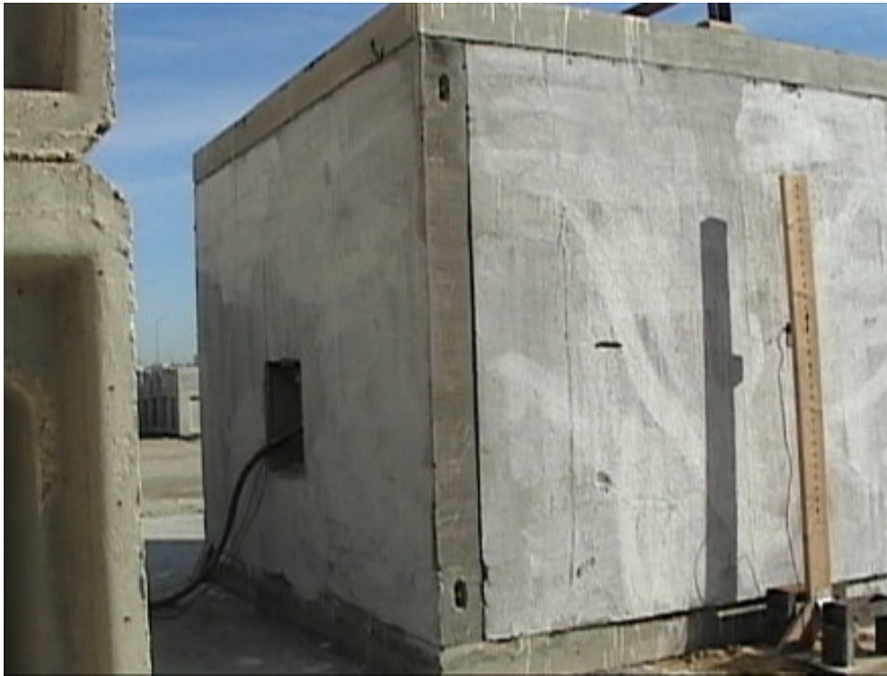
Figure 4.11 Building Prototype before Test No. 3
