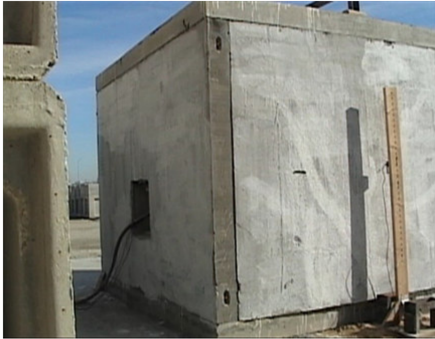
Figure 4.12 Building Prototype during Test No. 3 (Northwest Side)
