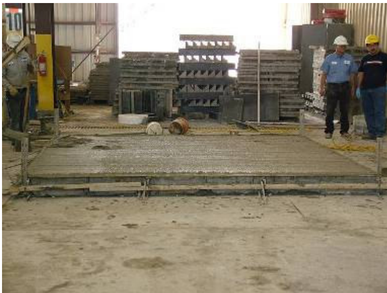
Figure A.12 Casting of Panels
