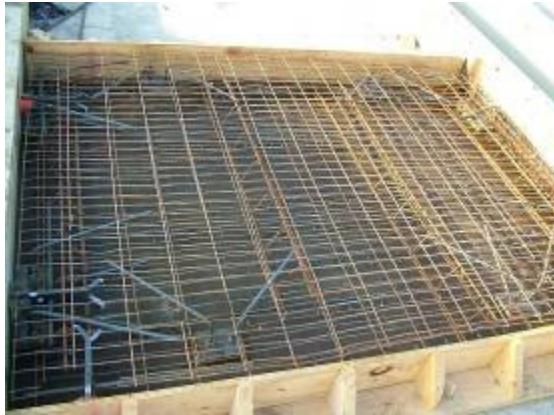
Figure 2.5 Formwork with Reinforcement
