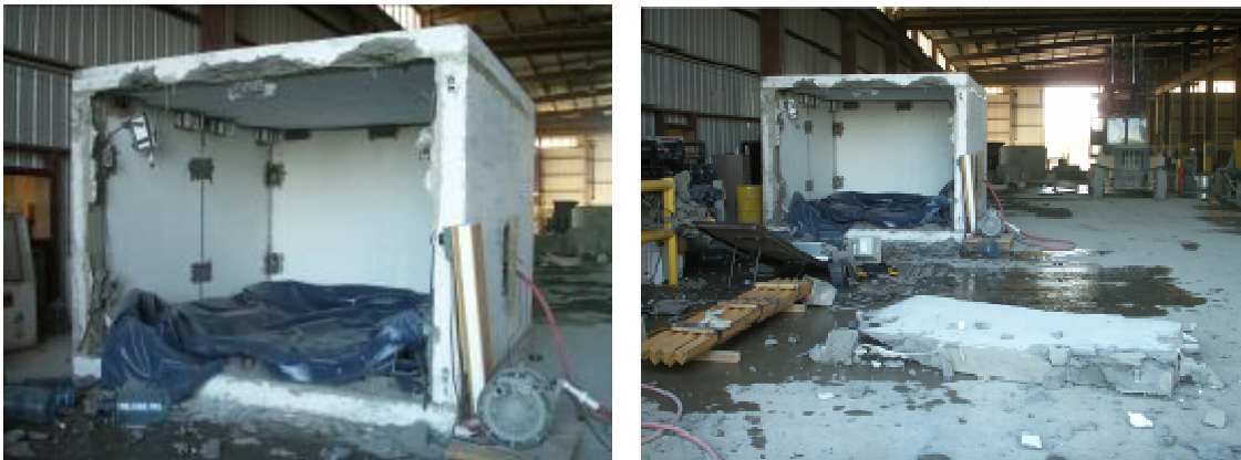
Figure 4.3 Building Prototype after Test No.1
