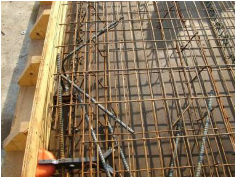
Figure A.8 Formwork with Wire Mesh
