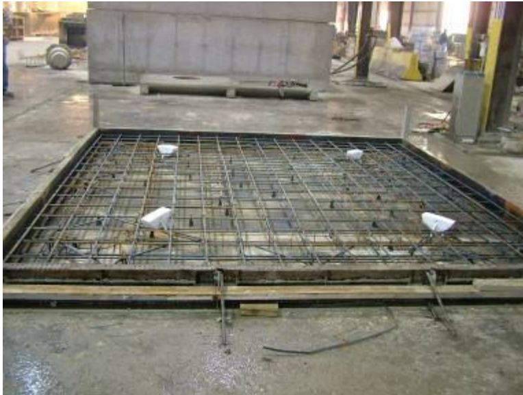
Figure A.3 Formwork for Panels
