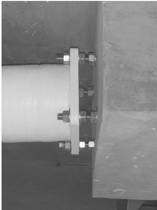
Figure 2.13 Bolt deformation at ultimate state
