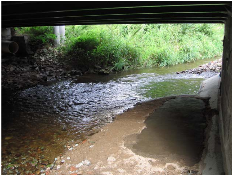
Figure 14. Experimental mud layer under the bridge on Bolíkovský stream.
